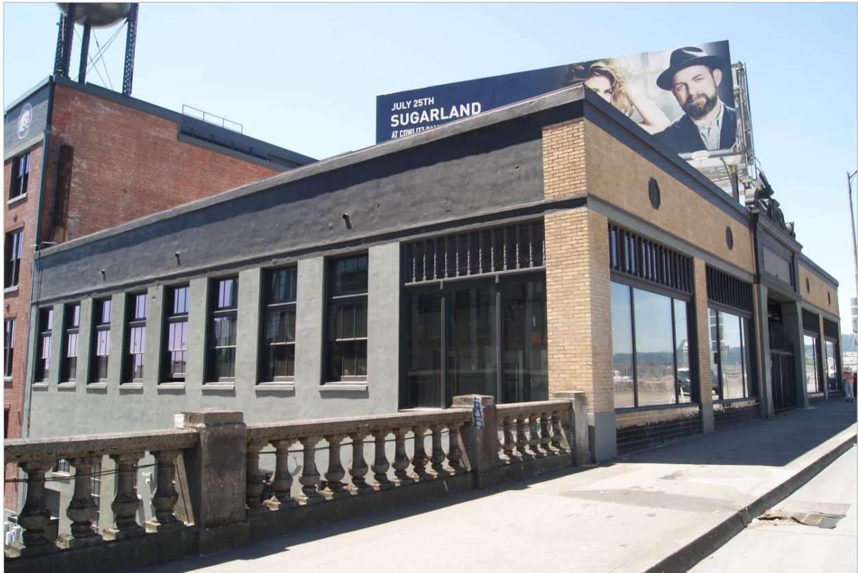
Figure 3.11-6. The Frigidaire/Templeton Building, looking west.
