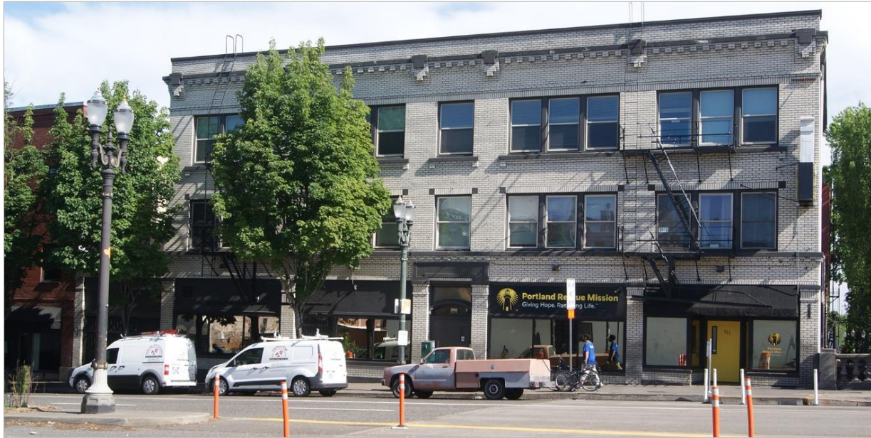
Figure 3.11-2. The Bates Building, looking north along West Burnside.
