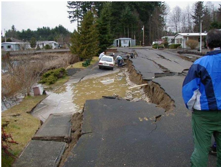
**Figure 4: Seismic Induced Ground Failure in Mw 9 Earthquake, Japan, 2011**
