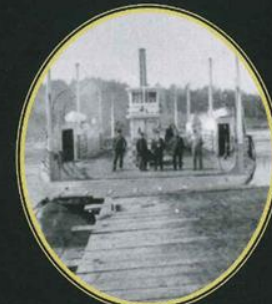
Ferryman John Ogden, "Carriage James Lee is in the center, Fred Galus, engineer is at the right." Portland, Oregon, 1904
