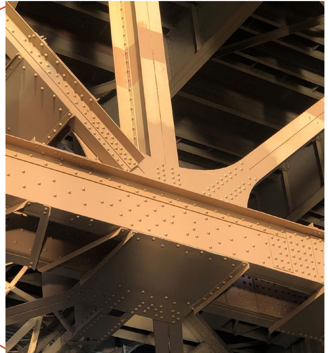
Approach Truss Node
