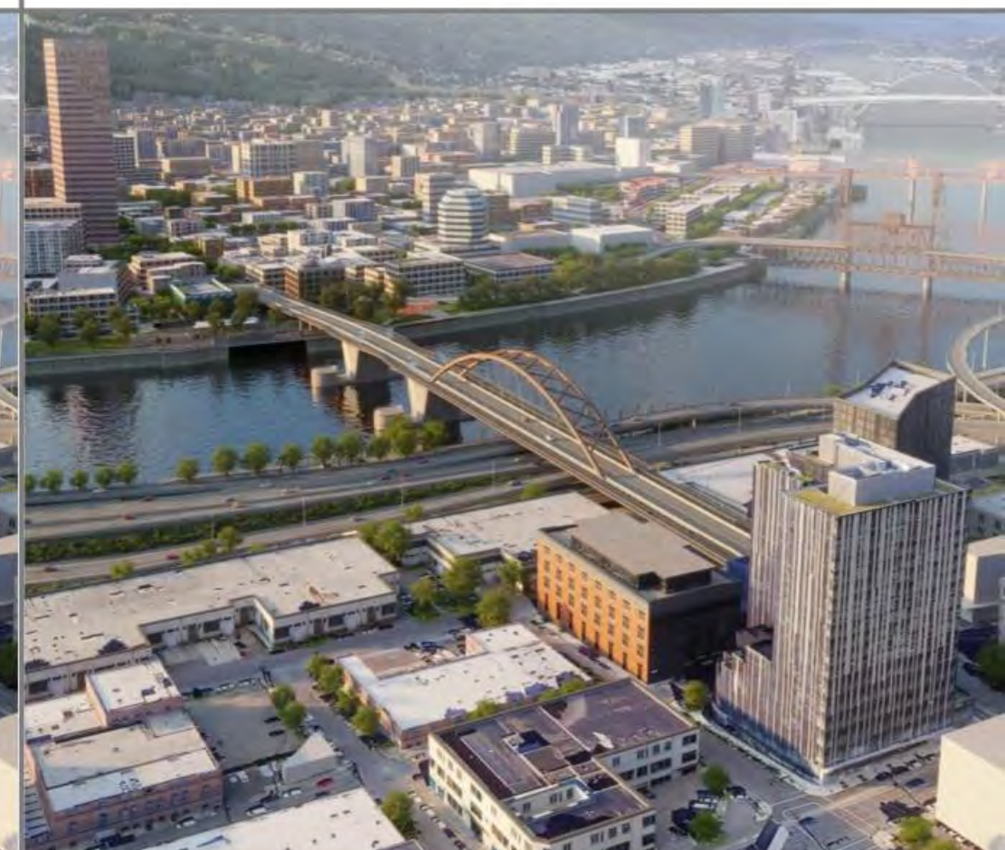
Tied-Arch Vertical Braced
