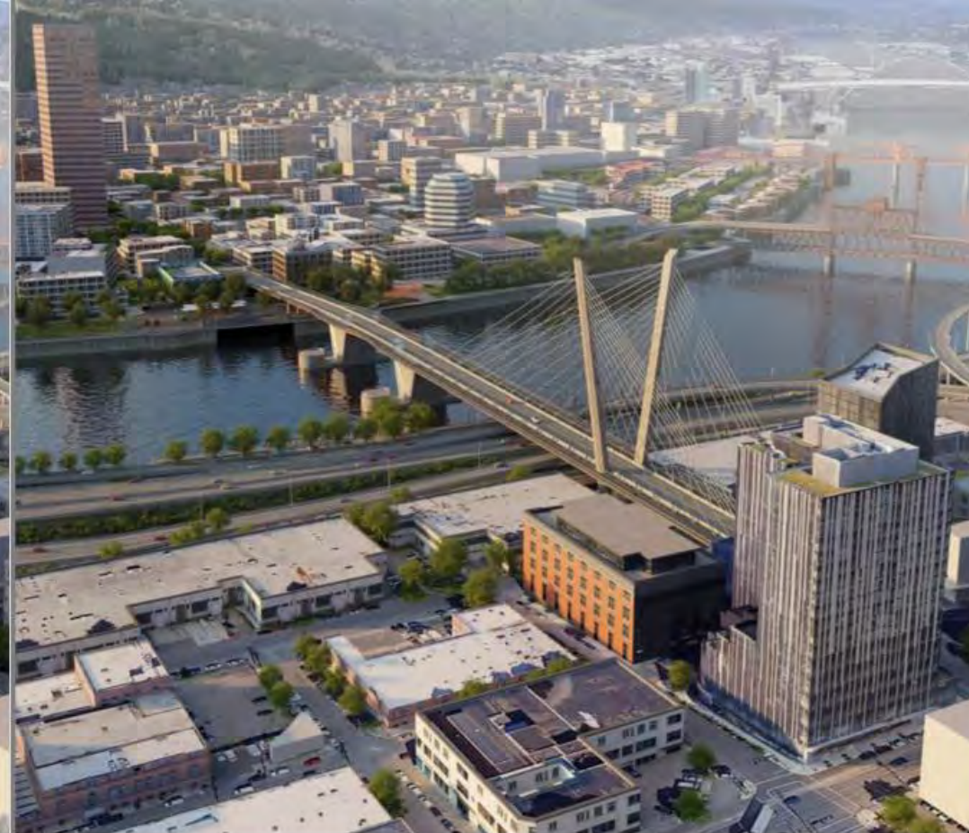
Cable-Stayed V Tower
