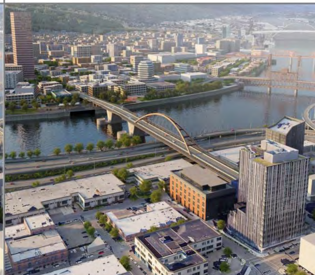
Tied-Arch Braced Basket Handle
