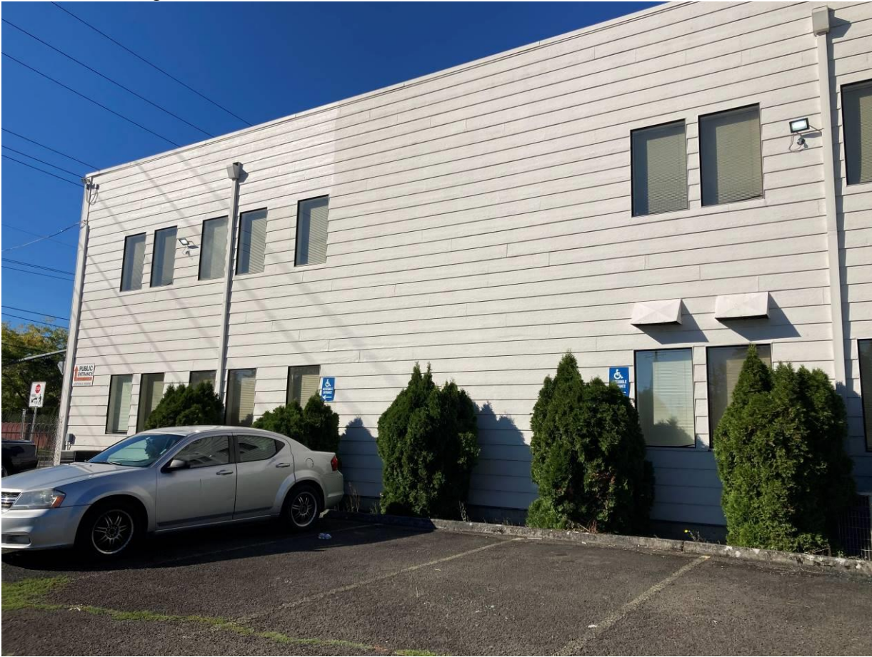
Photo 2. Building from the East
