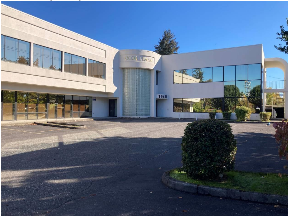
Photo 1. Existing Building from the Southwest
