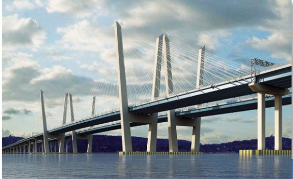
Cable Stayed / Extradosed
