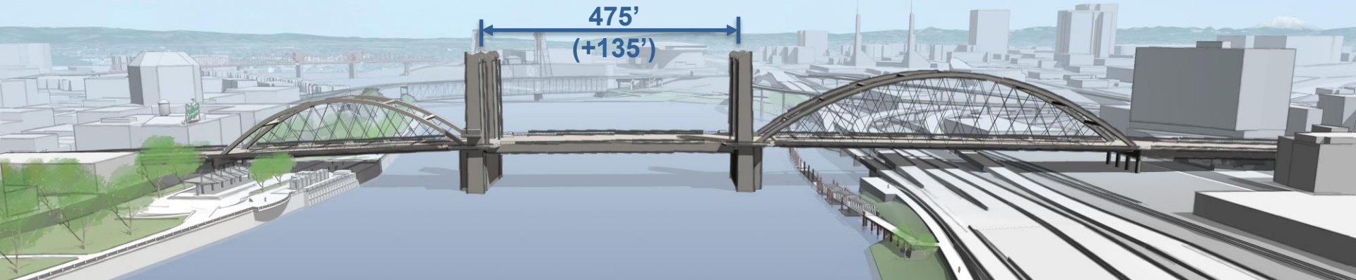
Long Movable Span (Tied Arch - Lift)
