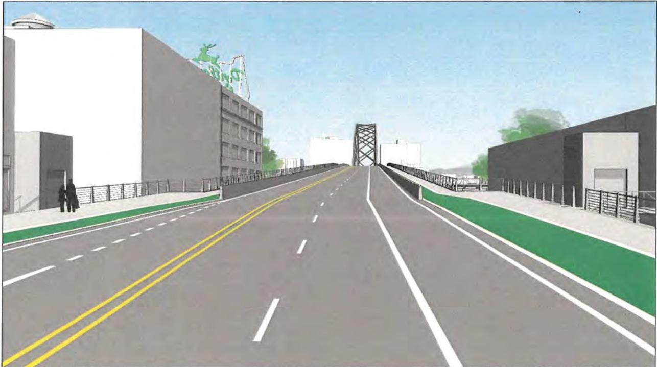
Figure 59: Span Combination 1 (girder west approach, bascule central span, tied arch east approach), artist's rendering, view looking east (Fat Pencil Studio, 2021). **NOTE: elevators omitted.**
