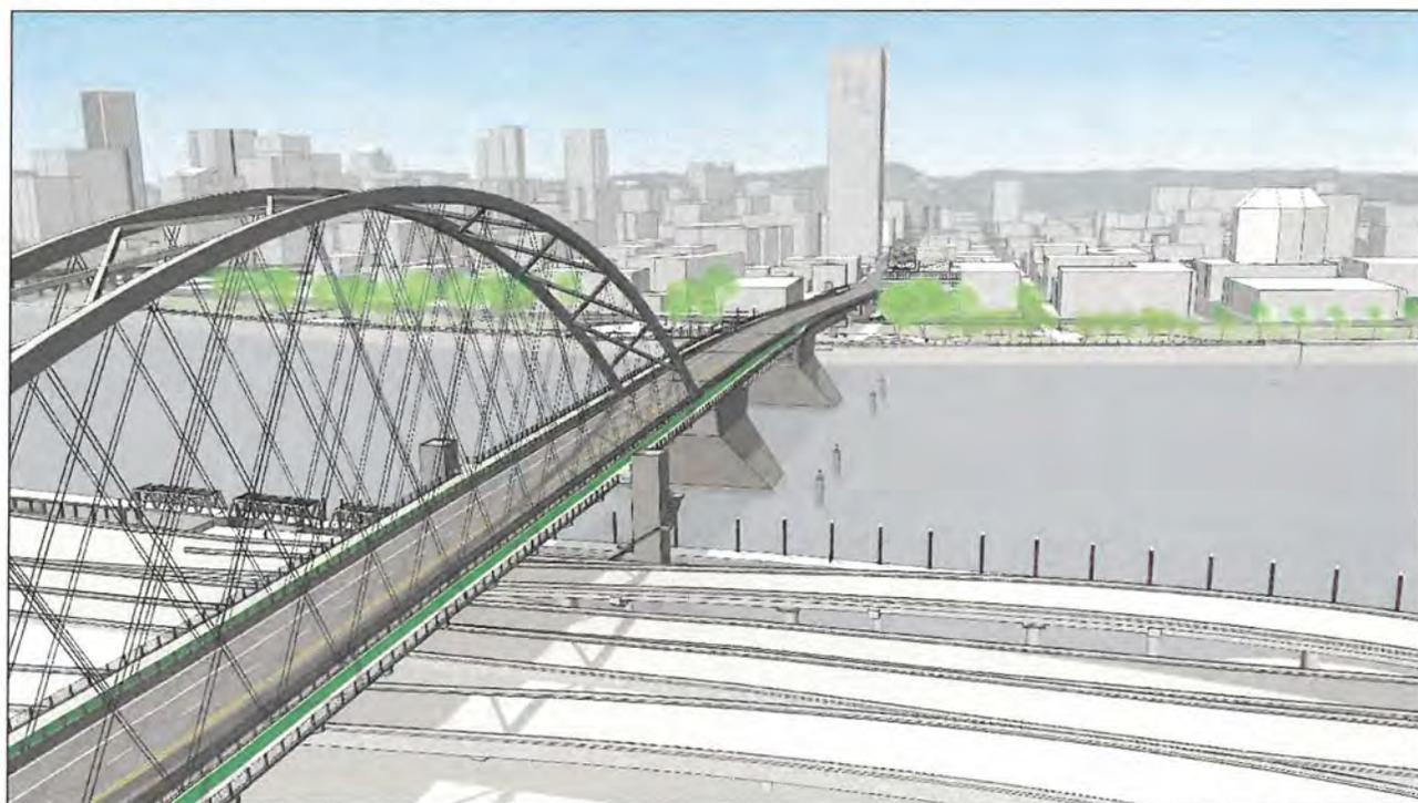
Figure 34: Span Combination 1 (girder west approach, bascule central span, tied arch east approach), artist's rendering, view looking southwest (Fat Pencil Studio, 2021).
