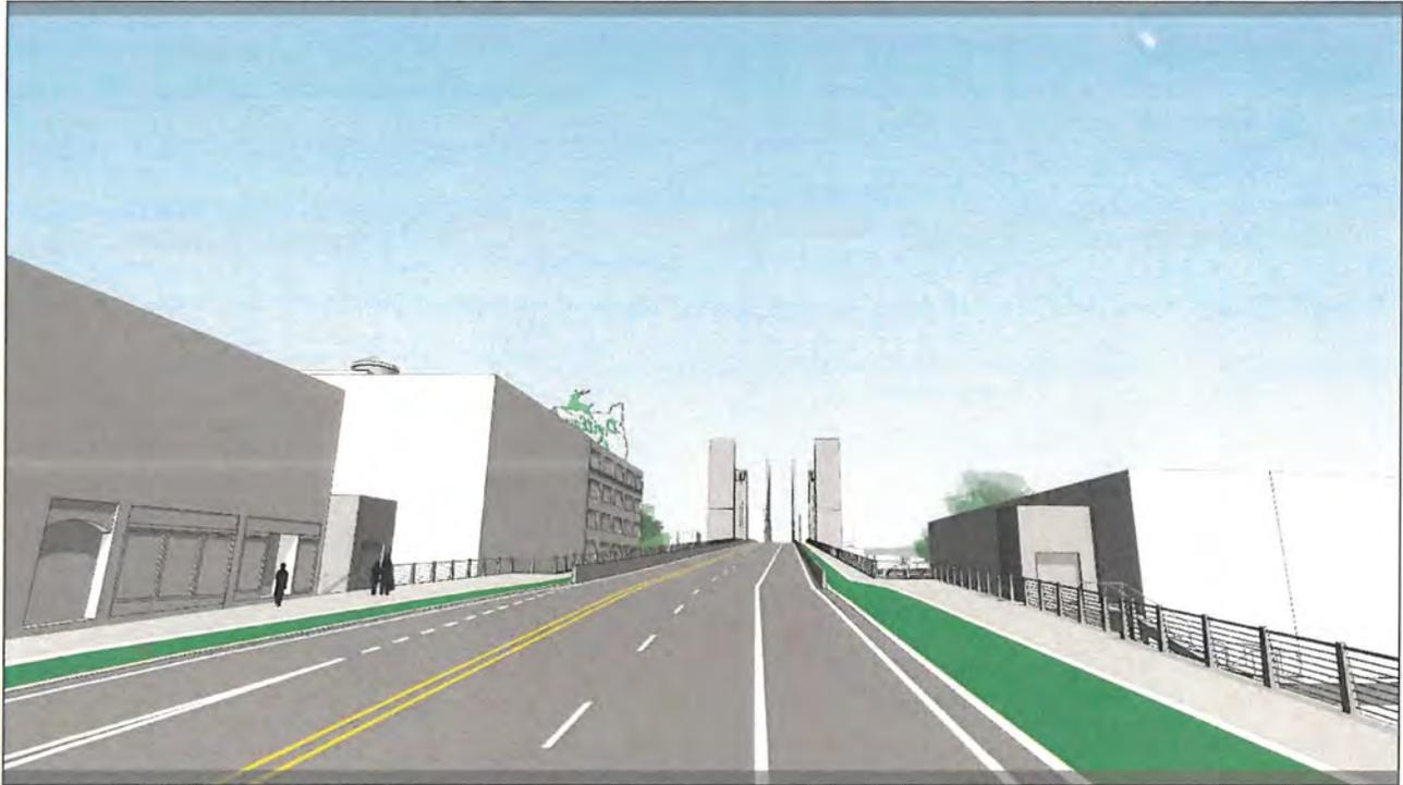
Figure 67: Span Combination 4 (girder west approach, vertical lift central span, cable supported east approach), artist's rendering, view looking east (Fat Pencil Studio, 2021). **NOTE: elevators omitted.**
