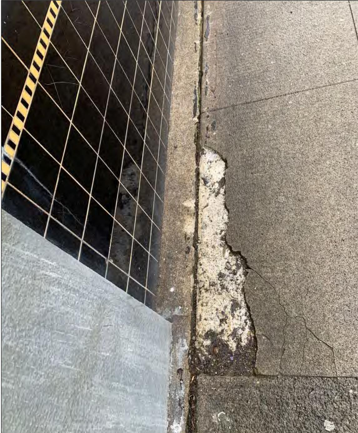
Figure 26: Frigidaire Building, detail view of cold joint between concrete ledger at north façade and sidewalk at east approach (Langston Guettinger, 2022).
