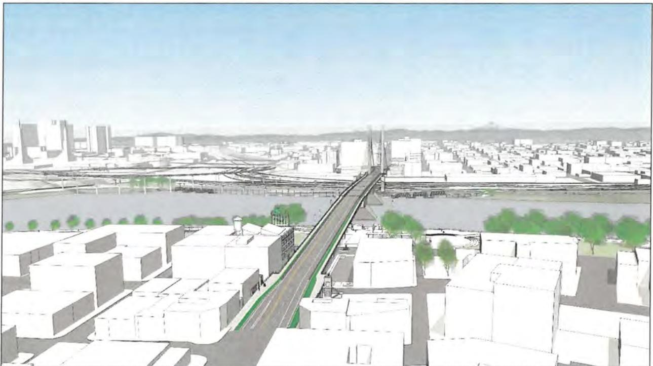
Figure 56: Span Combination 3 (girder west approach, bascule central span, cable supported east approach), artist's rendering, view looking east (Fat Pencil Studio, 2021). **NOTE: elevators omitted.**
