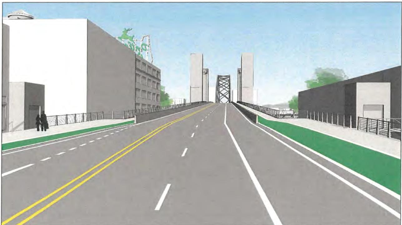
Figure 60: Span Combination 2 (girder west approach, vertical lift central span, tied arch east approach), artist's rendering, view looking east (Fat Pencil Studio, 2021). **NOTE: elevators omitted.**
