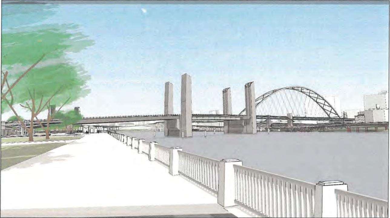
Figure 45: Span Combination 2 (girder west approach, vertical lift central span, tied arch east approach), artist's rendering, view looking north (Fat Pencil Studio, 2021).
