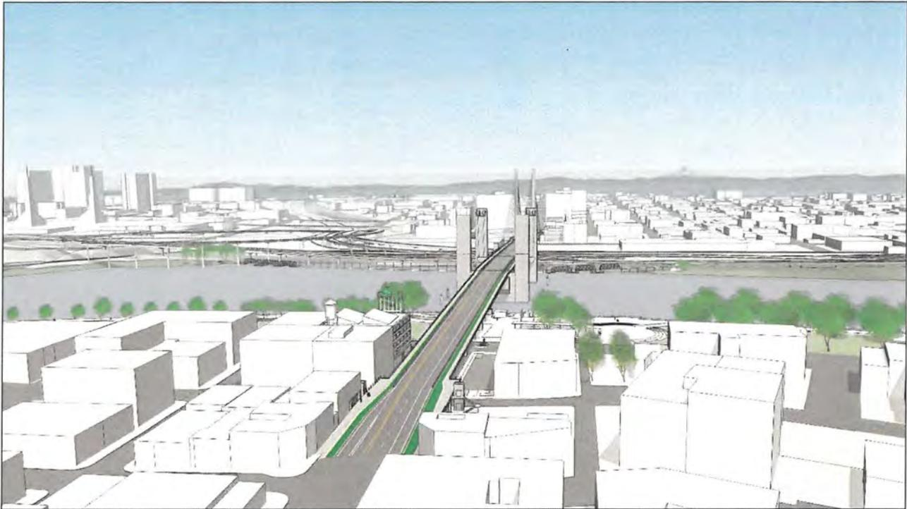
Figure 57: Span Combination 4 (girder west approach, vertical lift central span, cable supported east approach), artist's rendering, view looking east (Fat Pencil Studio, 2021). **NOTE: elevators omitted.**
