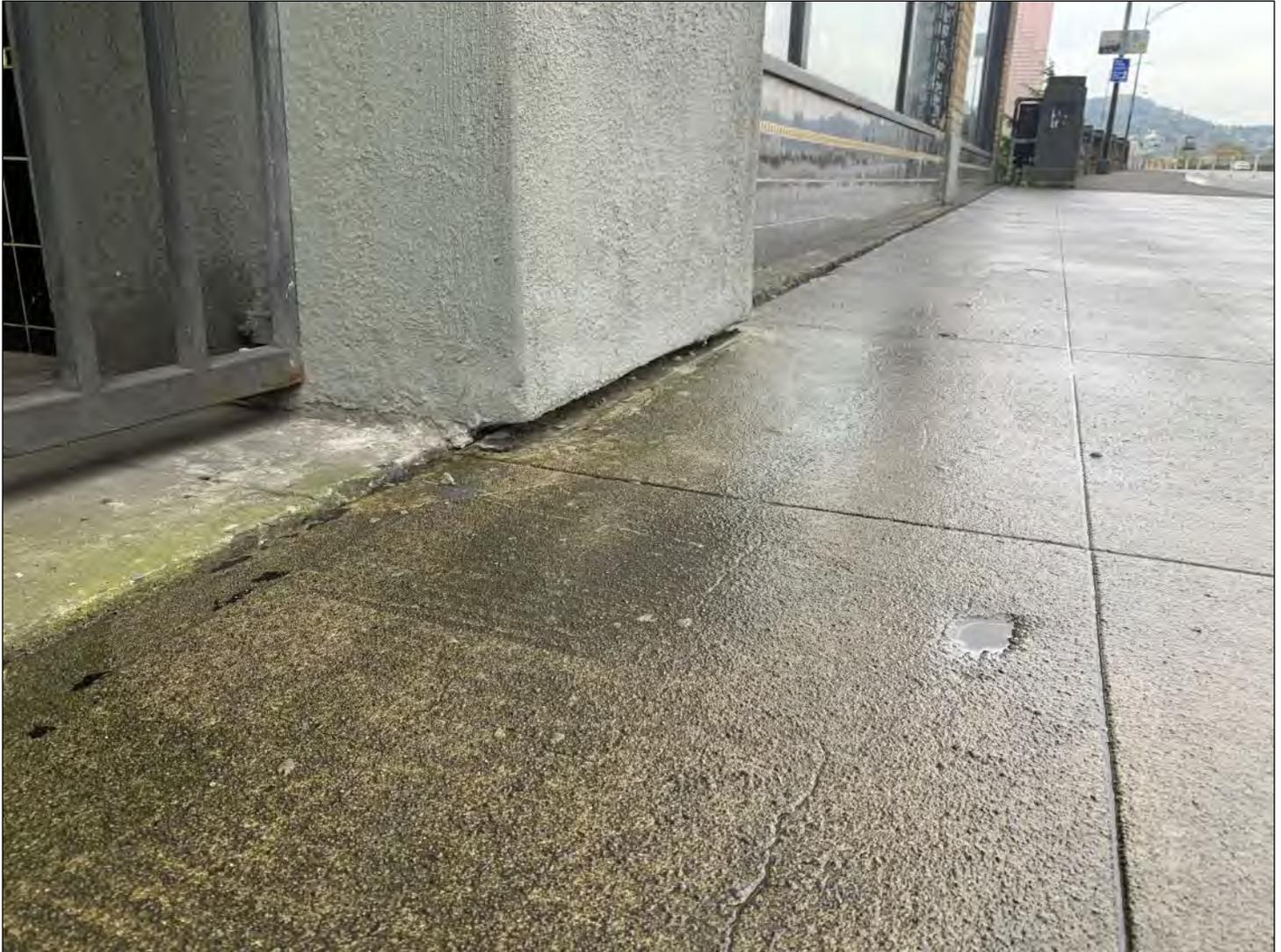
Figure 29: Frigidaire Building, detail view of cold joint between concrete ledger at north façade and sidewalk at east approach (Langston Guettinger, 2022).
