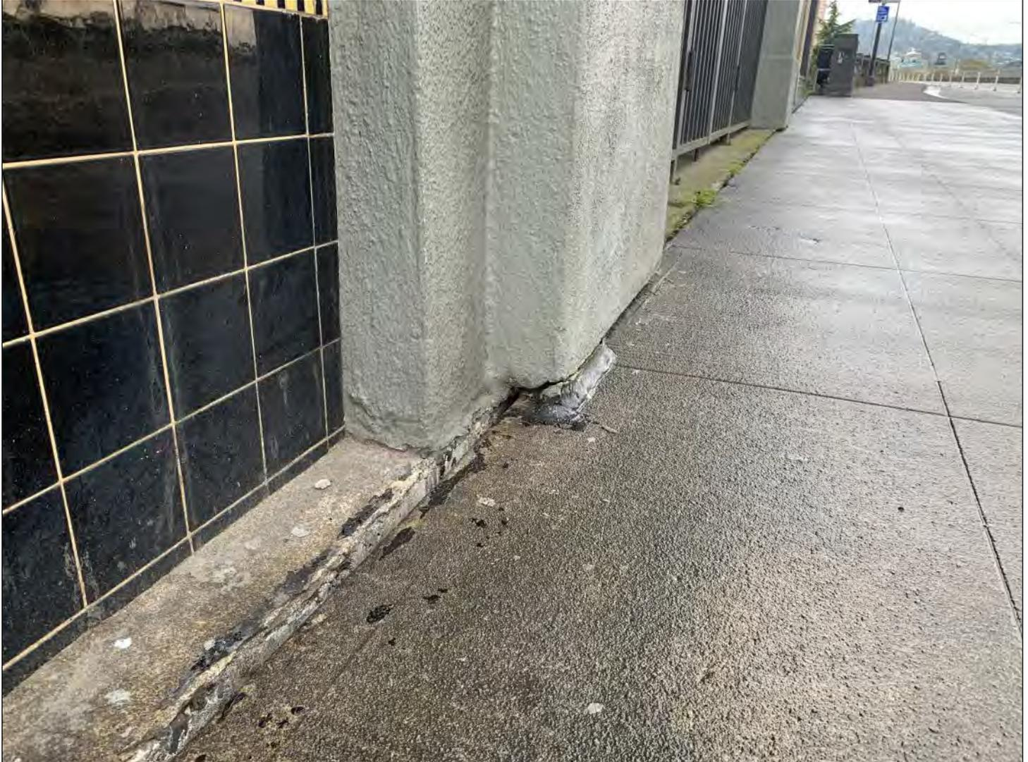
Figure 27: Frigidaire Building, detail view of cold joint between concrete ledger at north façade and sidewalk at east approach (Langston Guettinger, 2022).
