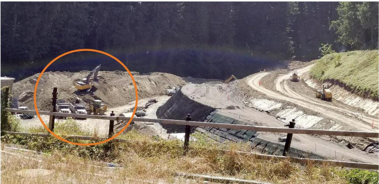
*Figure 7. Example of stockpile loading practices to reduce dust.*
