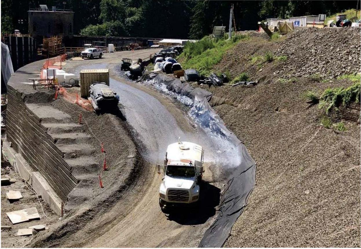
*Figure 6. Example of water truck pass to provide dust suppression on gravel construction roads.*
