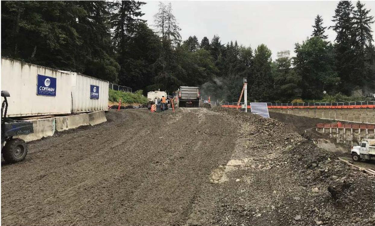
*Figure 2. Example of temporary gravel roads used for onsite construction vehicle traffic. Gravel roads produce less dust than dirt roads.*
