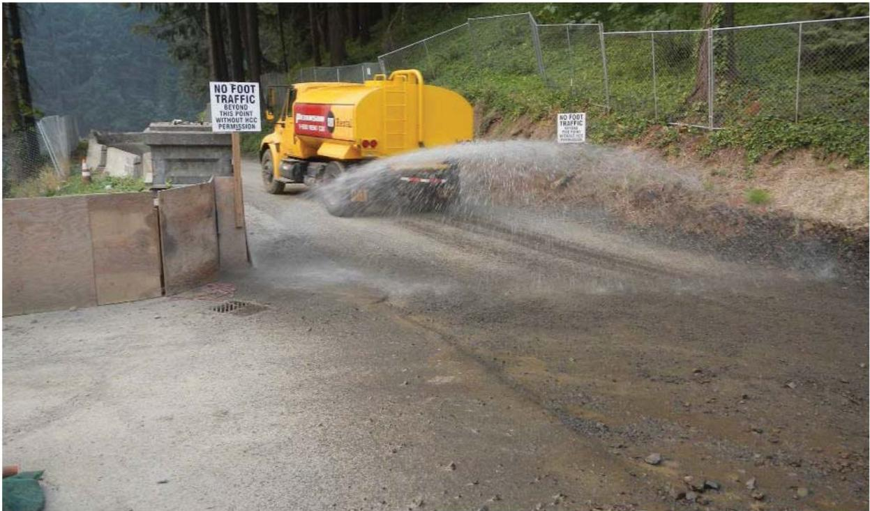
*Figure 5. Example of water truck pass to provide dust suppression on gravel construction roads.*
