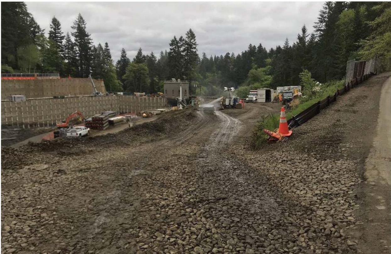
*Figure 3. Example of temporary gravel roads and larger construction entrance rock used for onsite construction vehicle traffic. Gravel roads produce less dust than dirt roads.*
