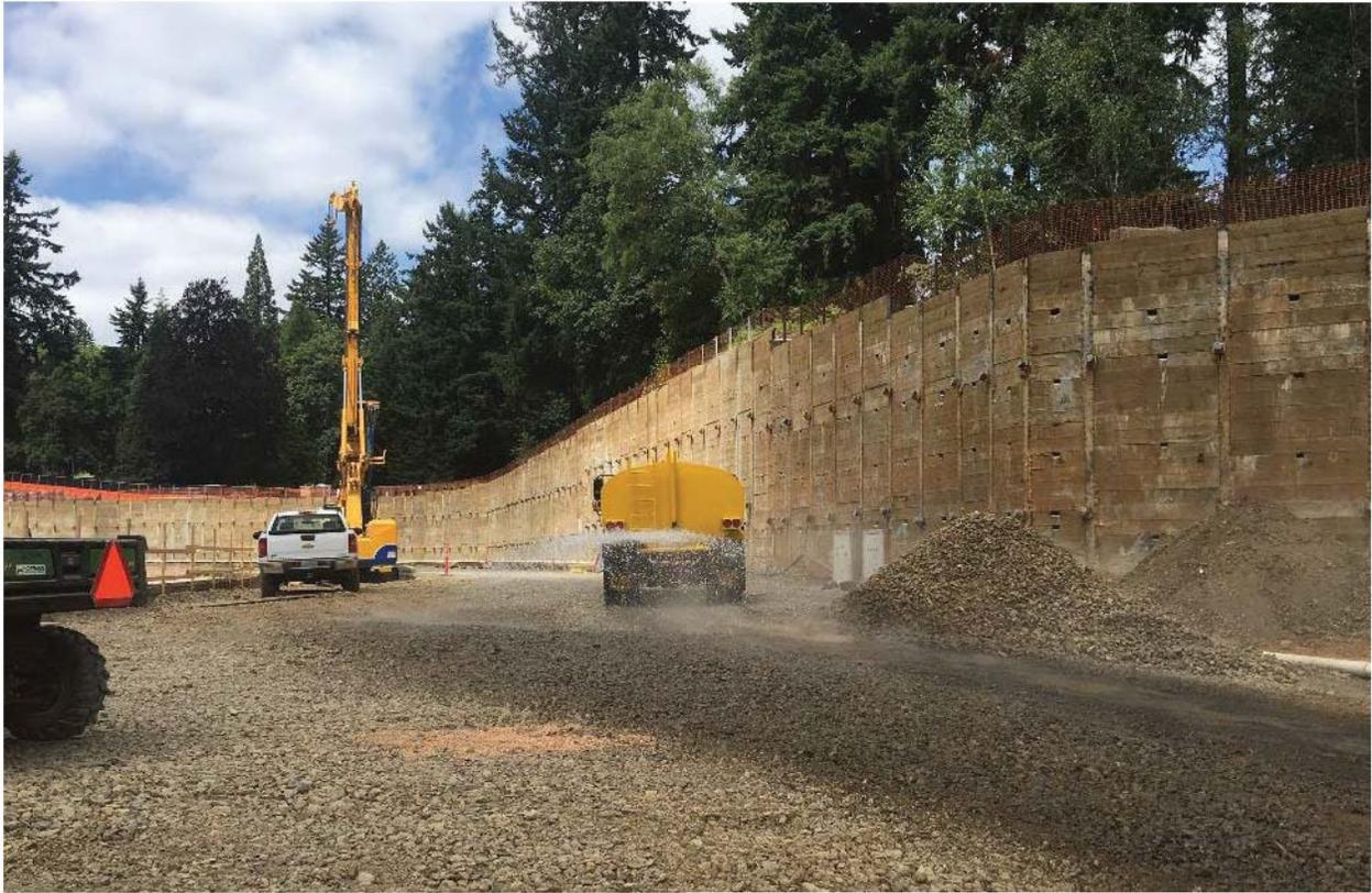
*Figure 4. Example of water truck pass to provide dust suppression on gravel construction roads.*
