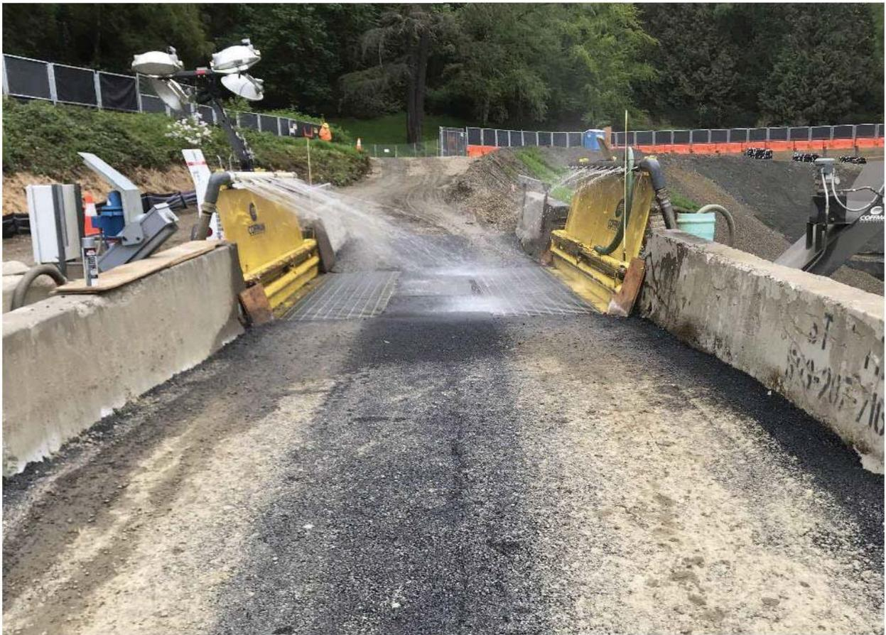
Figure 9. Example of wheel wash for construction vehicles leaving the site.
