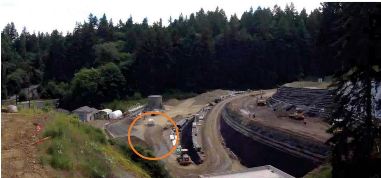
*Figure 1. Example of water truck pass to provide dust suppression on gravel construction roads.*
