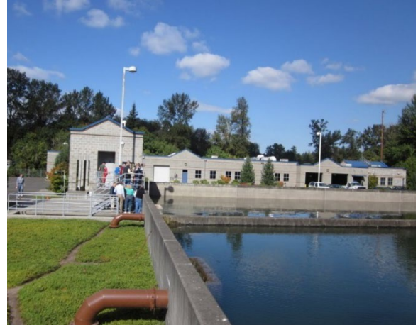
Photo of facility with basin in the foreground.
