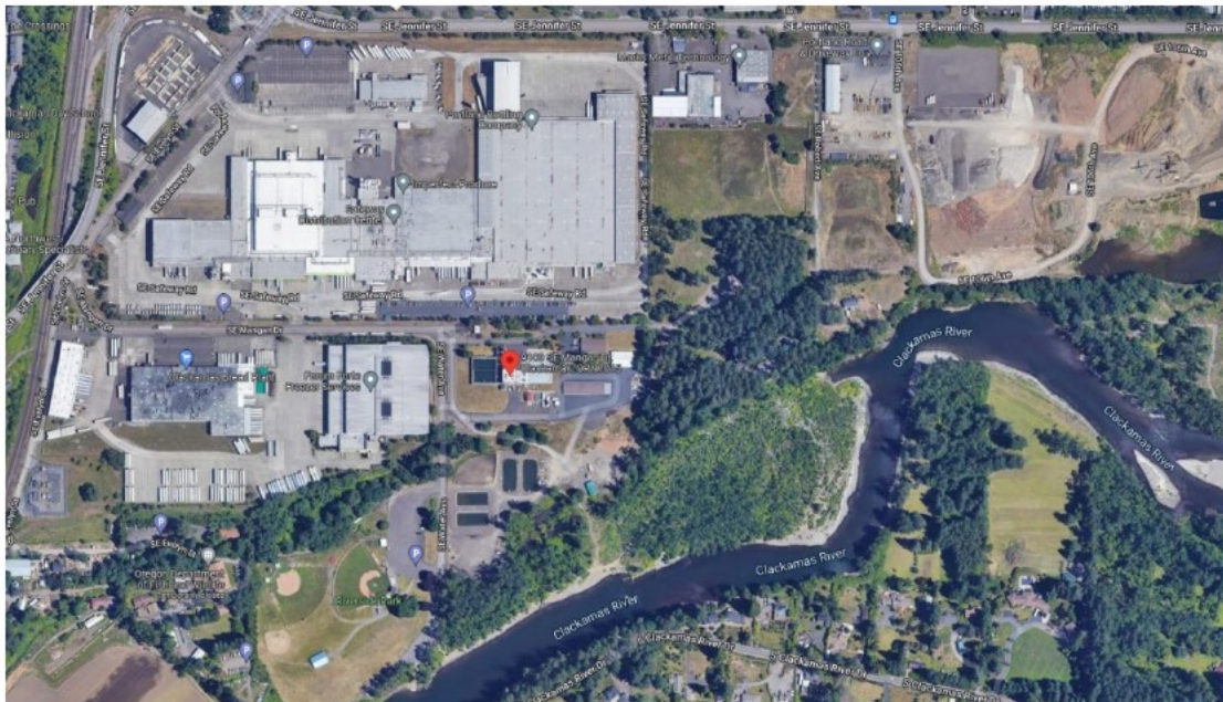
Aerial image showing location of the Clackamas River Water WTP near the Clackamas River.
