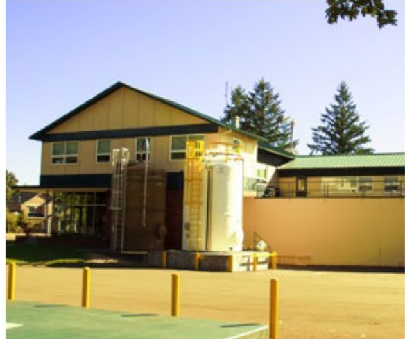
Photo of Collins Water Purification Works buildings.
