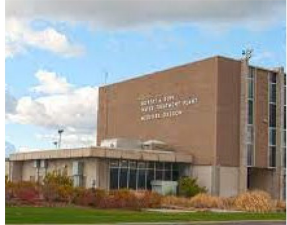
Photo of the Duff WTP buildings.
