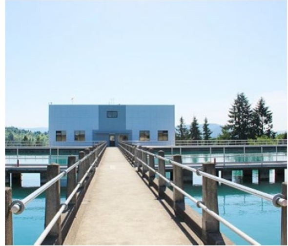
Photo of Hayden Bridge Water Filtration Plant with filters shown in foreground.
