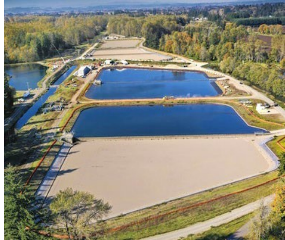
Photo of Geren Island WTP with view of filters and new ozone facility in background.
