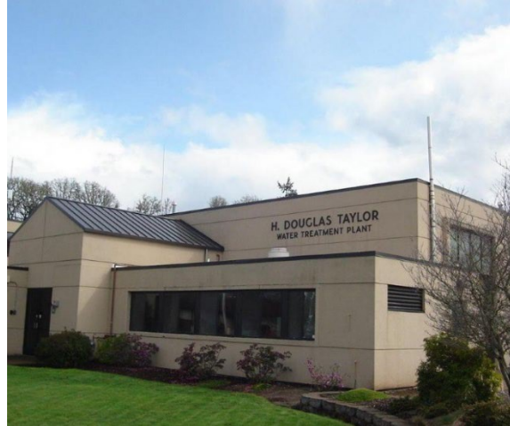
Photo of Taylor WTP buildings.
