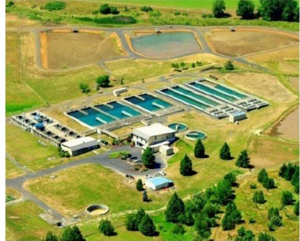
Aerial view of JWC WTP with view of basins.
