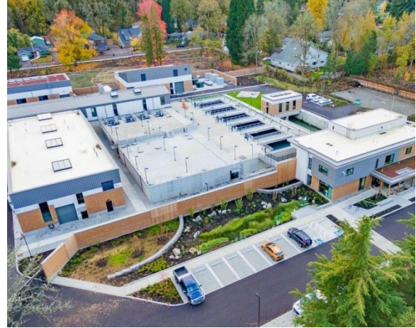
Photo of Lake Oswego-Tigard WTP.
