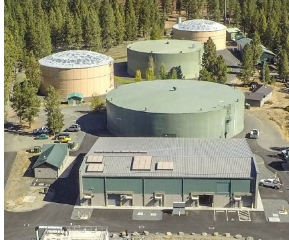
Photo of facility with storage reservoirs in the background.
