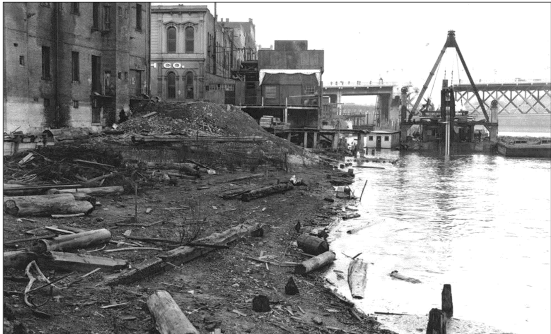
Figure A-5. Clearance of Docks and Wharves in Preparation of Construction of the Harbor Wall, with the Burnside Bridge to the North. Photo dated January 31, 1928.
