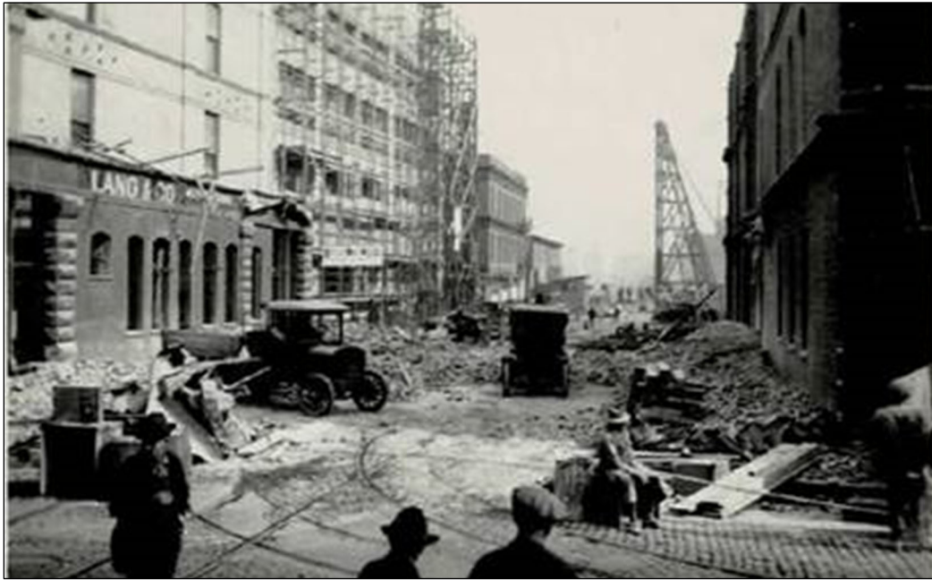
Figure A-11. Photograph of the Widening of Burnside
