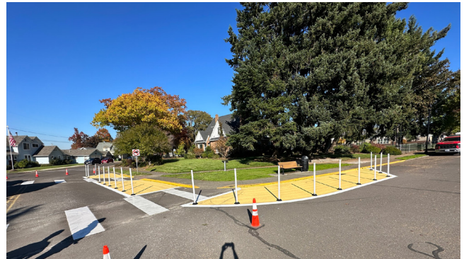
Modular curb protected bike lane
