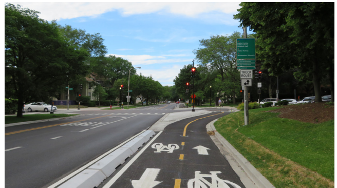
Modular curb protected bike lane
