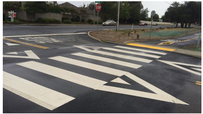
Advance stop bar and high visibility crosswalk
