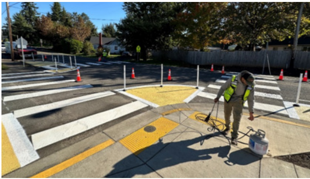
Painted curb and bollard curb extensions
