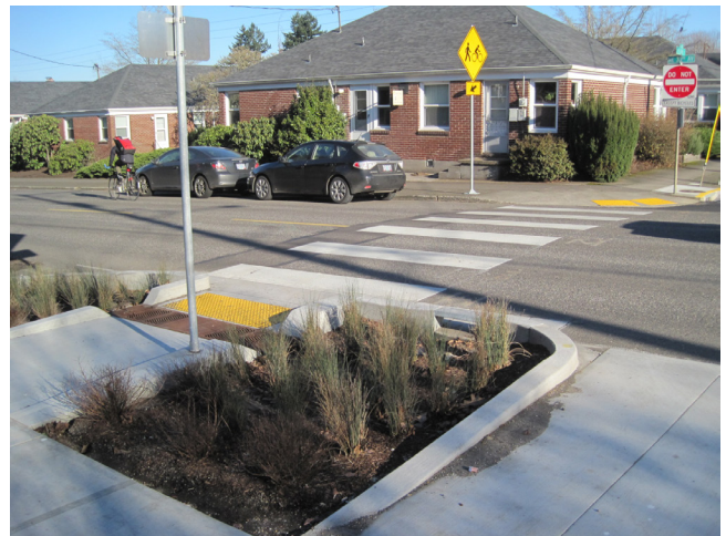
Enhanced crosswalk (above) and curb extension (below)
