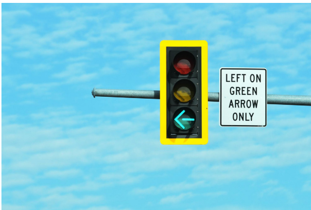
Protected or protected/permissive left turn phasing
