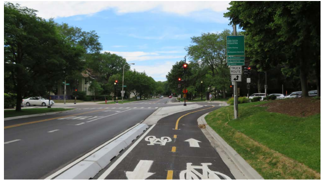
Modular curb protected bike lane
