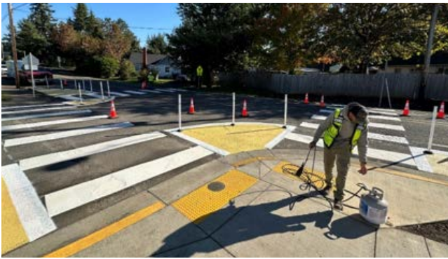
Painted curb and bollard curb extensions
