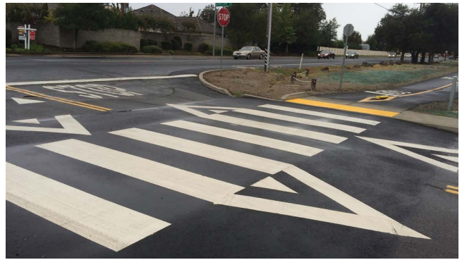
Advance stop bar and high visibility crosswalk
