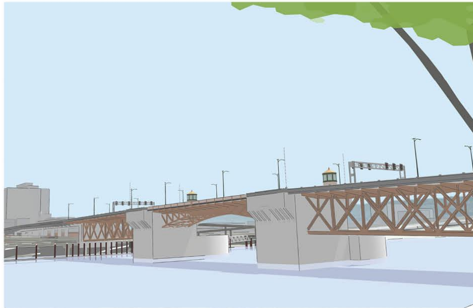
Enhanced Seismic Retrofit Alternative
