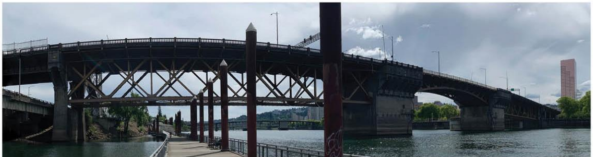
7. View from Vera Katz Eastbank Esplanade floating walkway looking south
