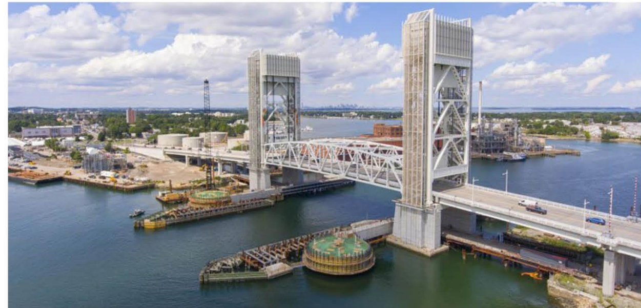
Fore River Bridge, Quincy, Massachusetts
