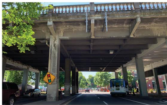
6. Burnside Bridge from Naito Pkwy looking south
