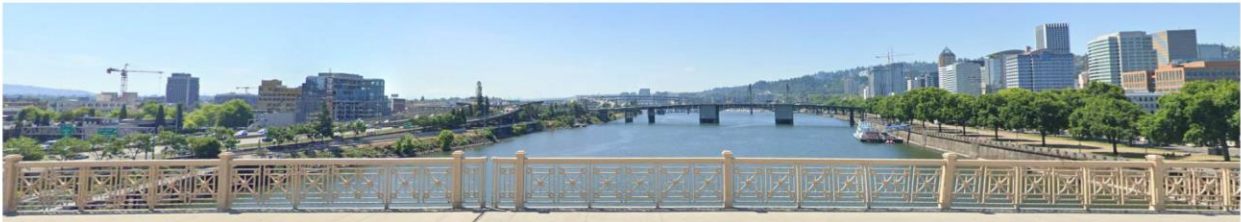
8. CCSE01: Burnside Bridge - South Side, Center
