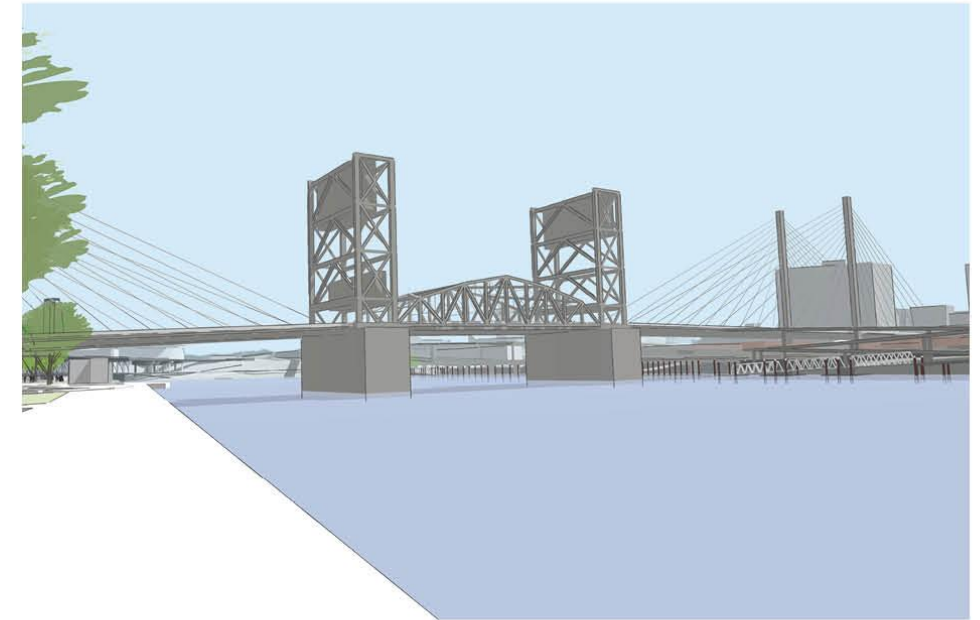
Long-span Alternative / Cable-stayed / Lift
