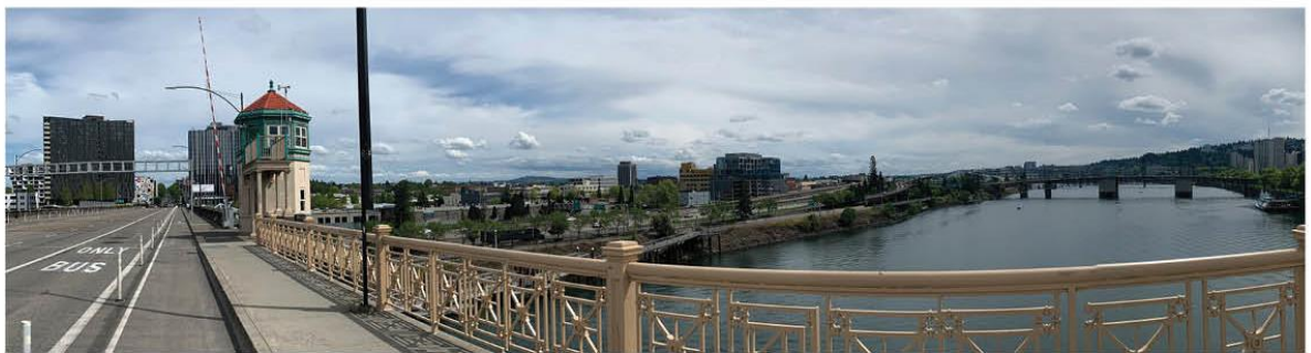
3. View from Burnside Bridge looking southeast
