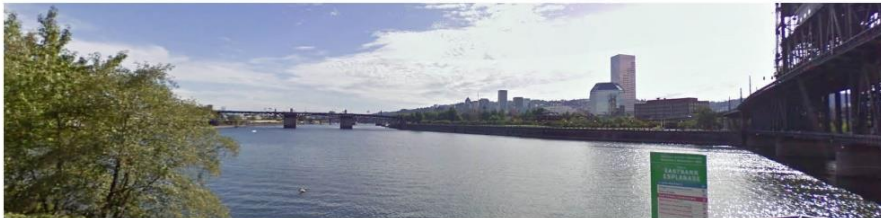
3. CCNE06: Mid-Ramp on Bike/Pedestrian Path to Steel Bridge
