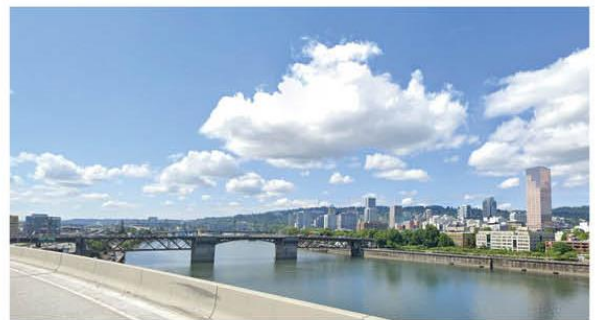
6. View from I-5 ramp looking southwest
