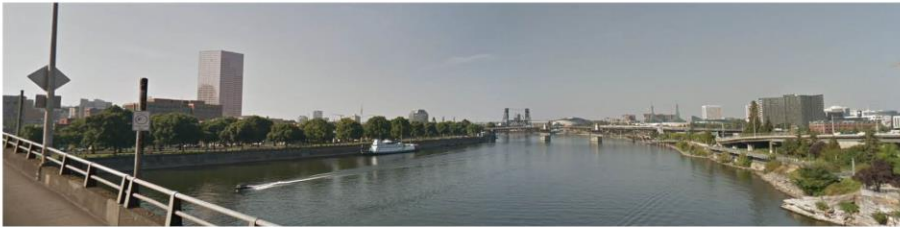
7. CCSE06: Morrison Bridge - North Side, East
