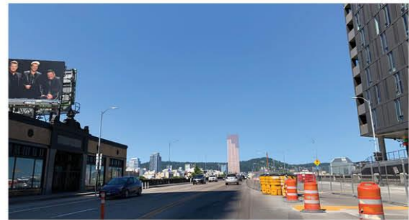
2. View from E Burnside Street to Burnside Bridge looking west
