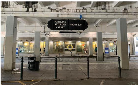
4. Skidmore Fountain MAX Station on 1st Ave under Burnside Bridge looking west
