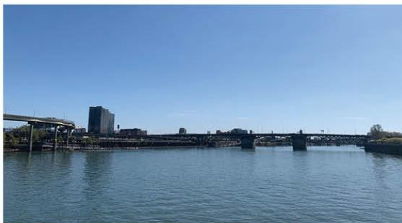
5. View from Steel Bridge looking south
