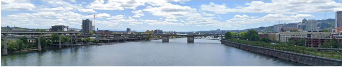
1. CCNW20: Steel Bridge - South Side (Upper Deck), Center
