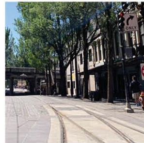
Light rail tracks
