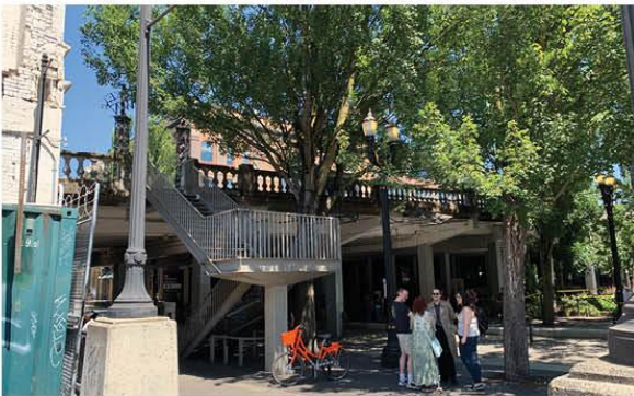
3. Pedestrian stair at SW 1st Ave looking northeast
