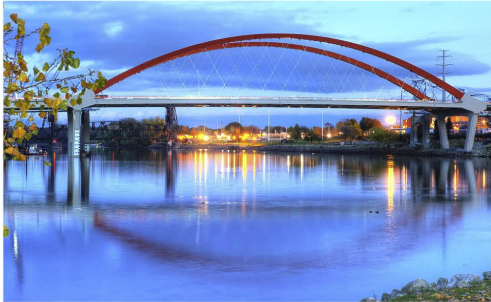
Hastings Bridge, Hastings, Minnesota
