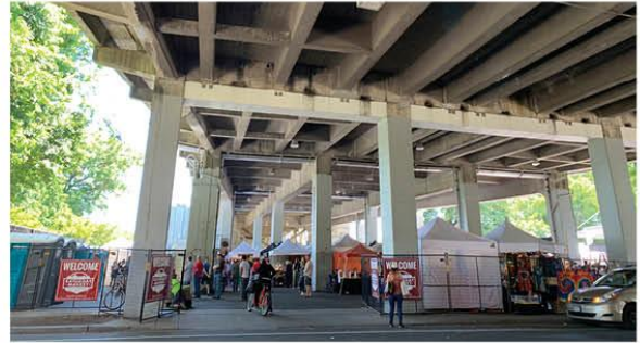
11. View from Naito Parkway under Burnside Bridge looking east
