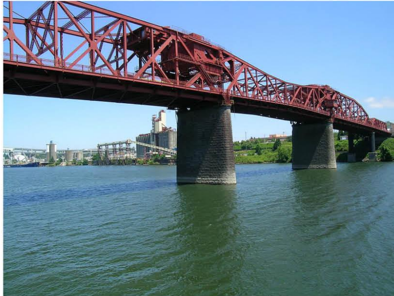
Broadway Bridge, Portland, Oregon
