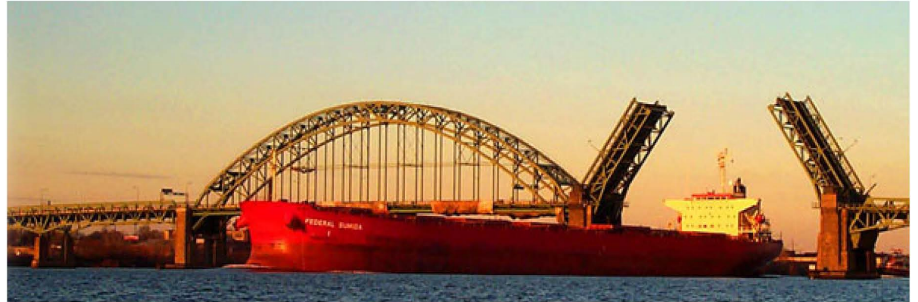
Tacony-Palmyra Bridge, New Jersey
