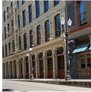
Standard acorn lights and typical building facade
