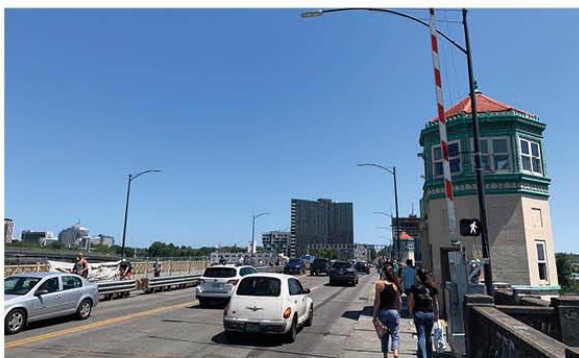
8. Burnside Bridge deck looking east - not lifted
