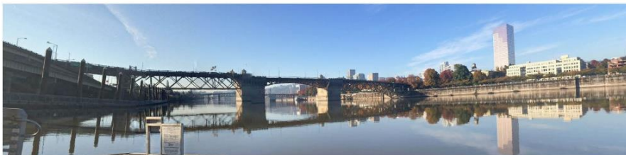
4. CCNE10: Duckworth Dock - South End
