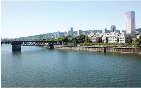
13. Burnside Bridge and Downtown from Steel Bridge looking south
