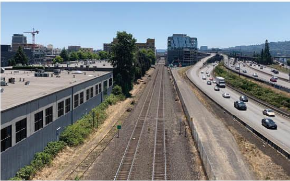
19. Union Pacific Railroad from Burnside Bridge looking south
