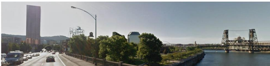
5. CCNE11: Burnside Bridge - North Side, Center
