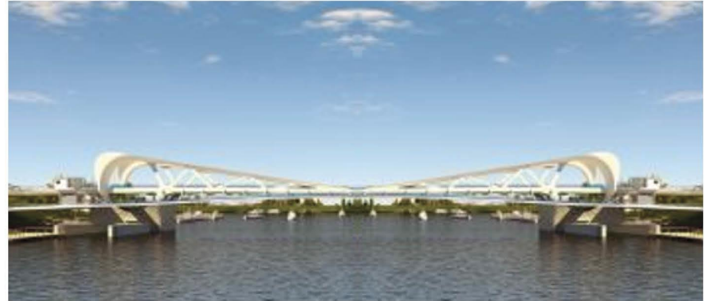
New Johnson Street Bridge, Victoria, Canada
