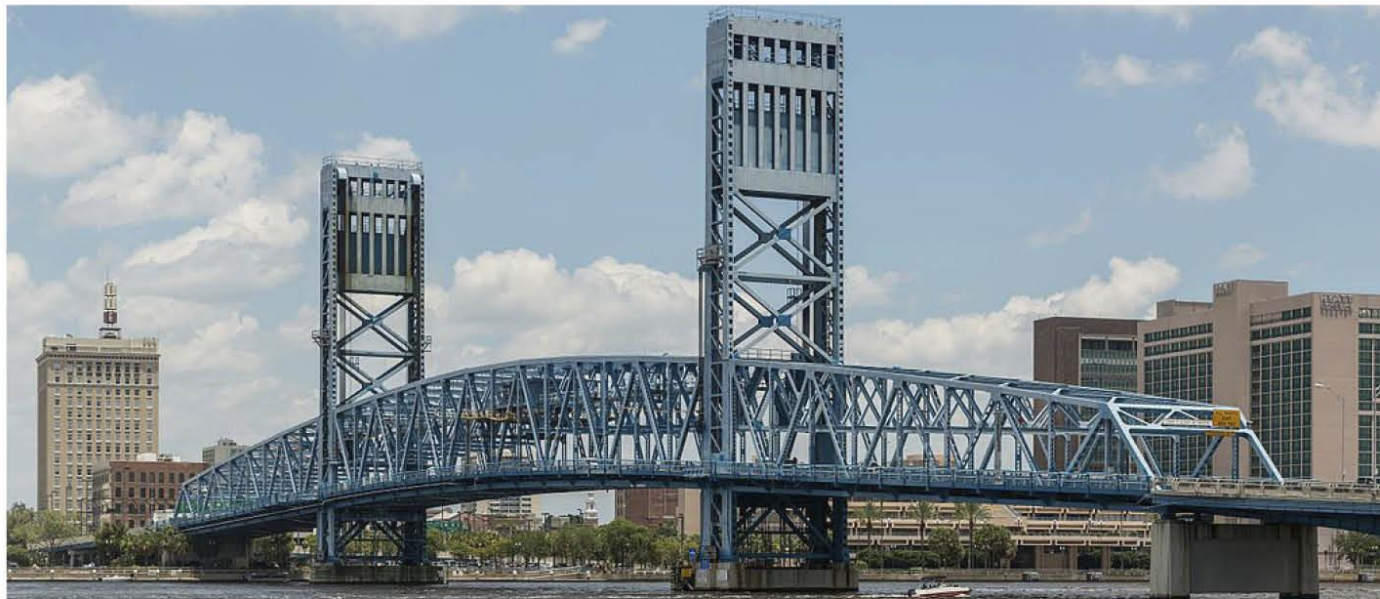
Main Street Bridge, Jacksonville, Florida
