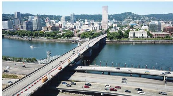
1. View from Eastside to Burnside Bridge looking west
