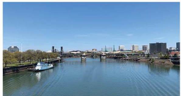
9. View from Morrison Bridge looking north
