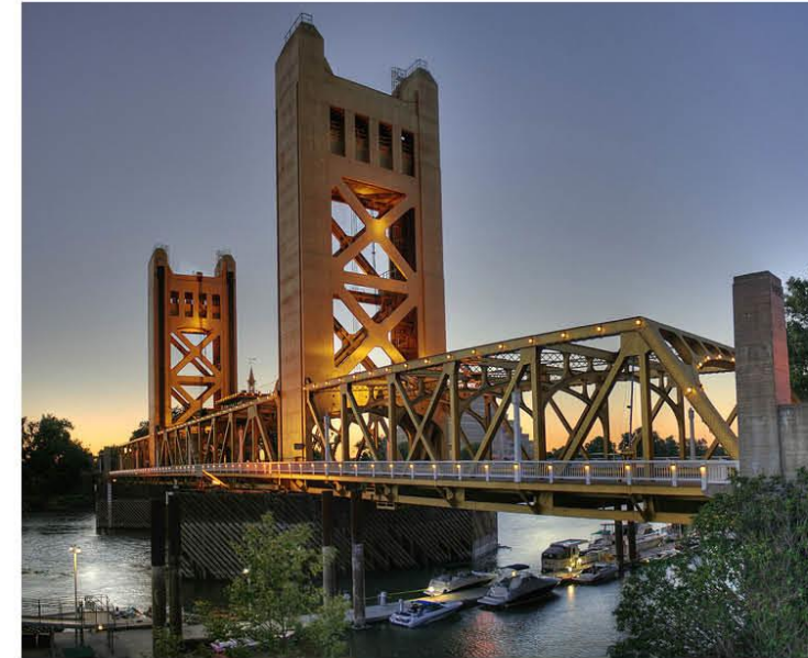
Tower Bridge, Sacramento, California
