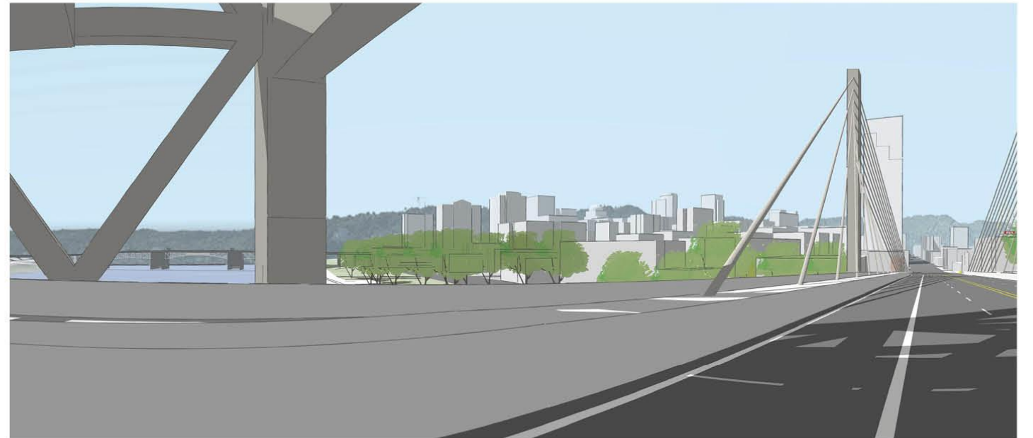
Long-span Alternative / Cable-stayed / Lift
