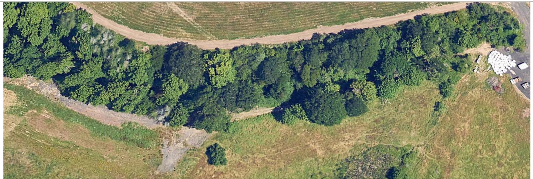
06/27/2023 Closeup of Southern Portion of Road A
