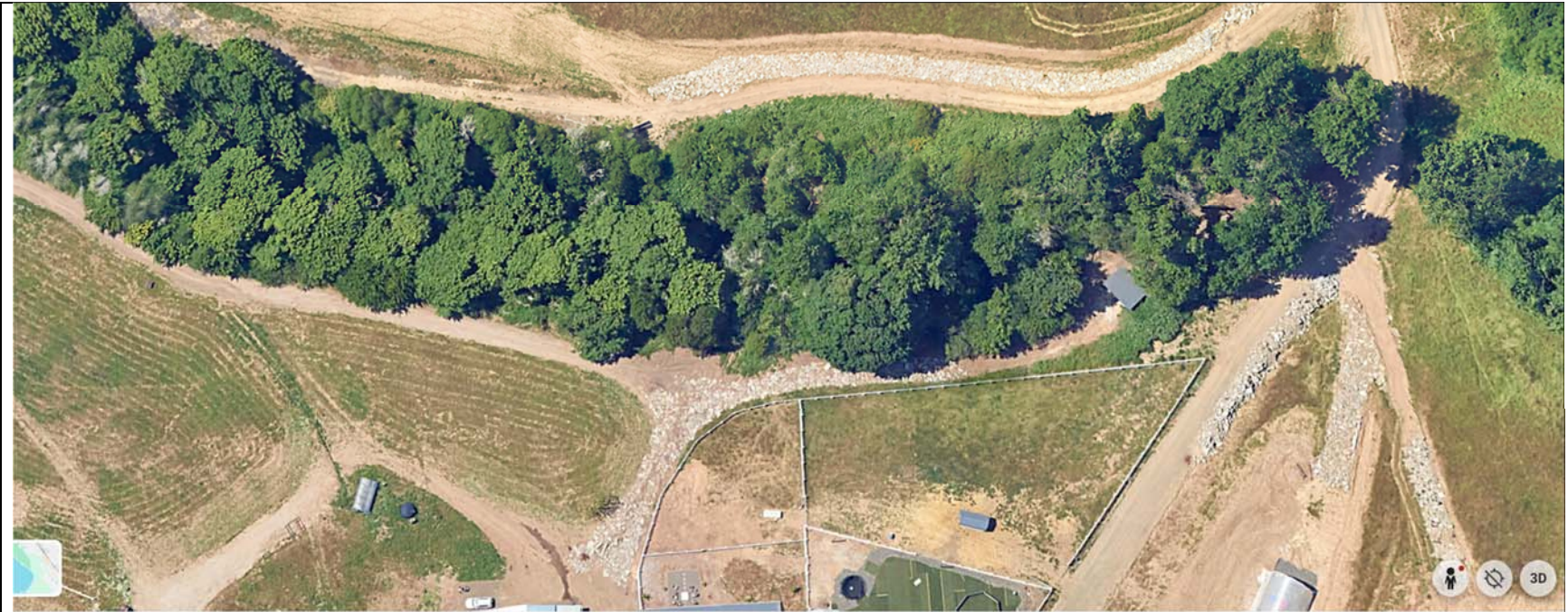
06/27/2023 Closeup of Northern Portion of Road B
