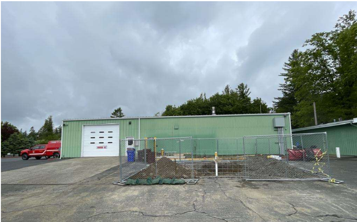
Figure 7: South elevation of Corbett Fire Station. View 312°. Photo taken on 05/12/2025.
