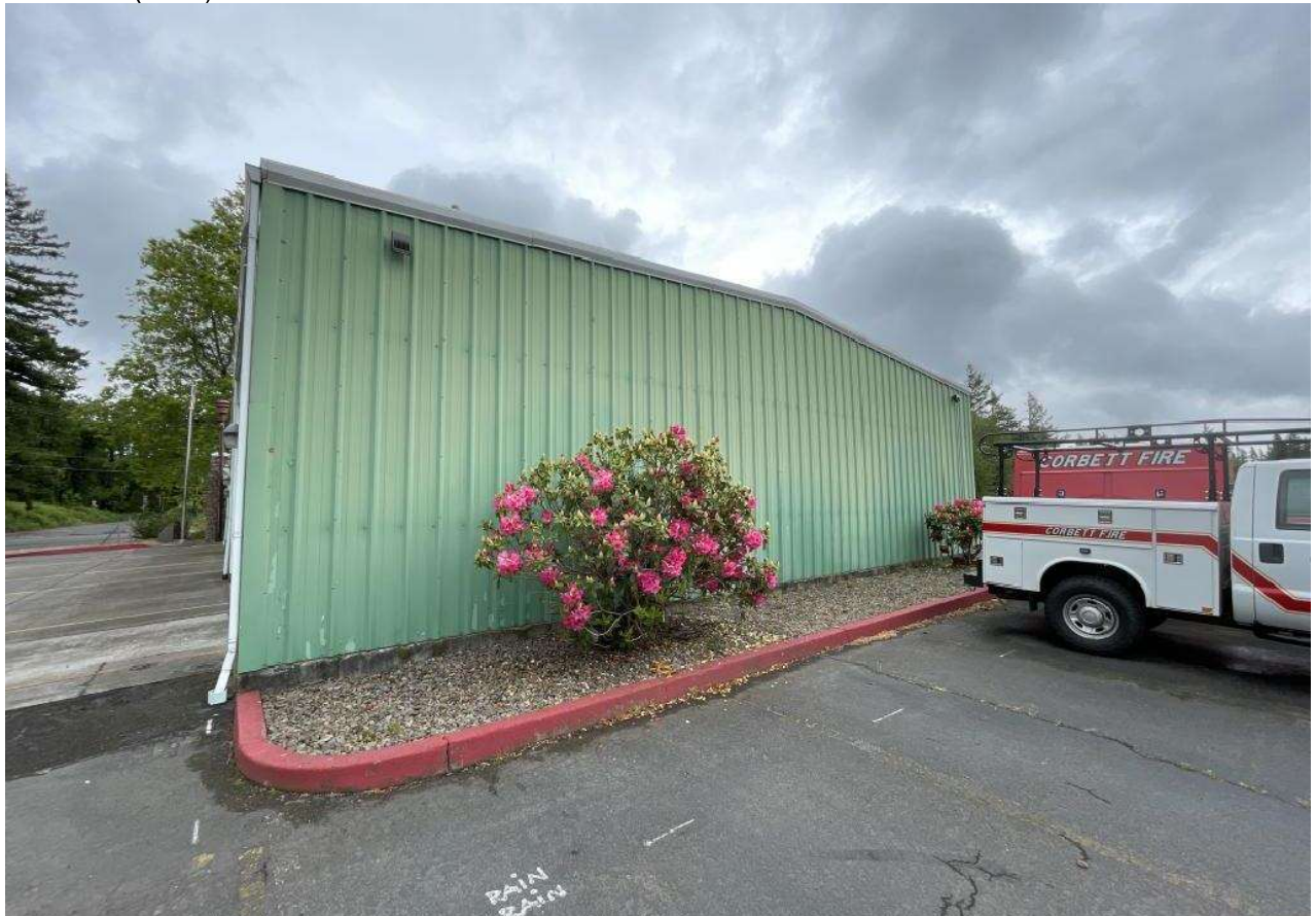
Figure 5: West elevation of Corbett Fire Station. View 148°. Photo taken on 05/12/2025.
