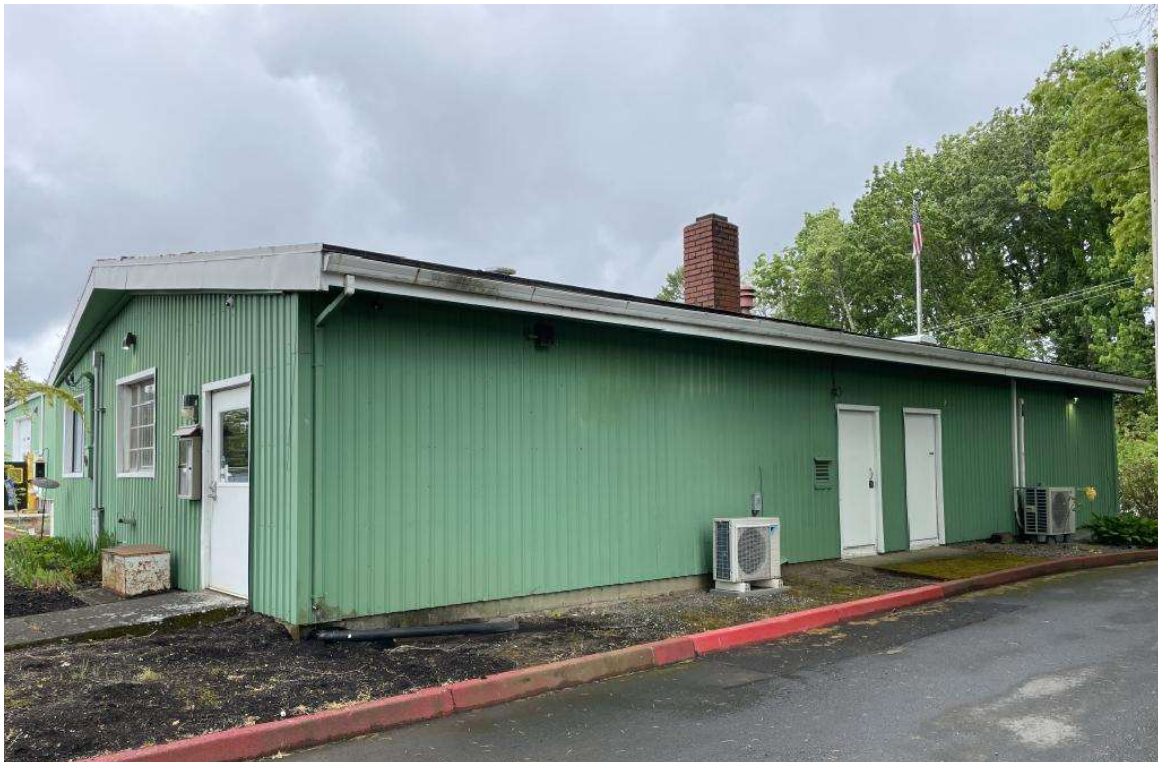
Figure 11: East elevation of the Corbett Fire Hall. View 289°. Photo taken 5/12/2025.
