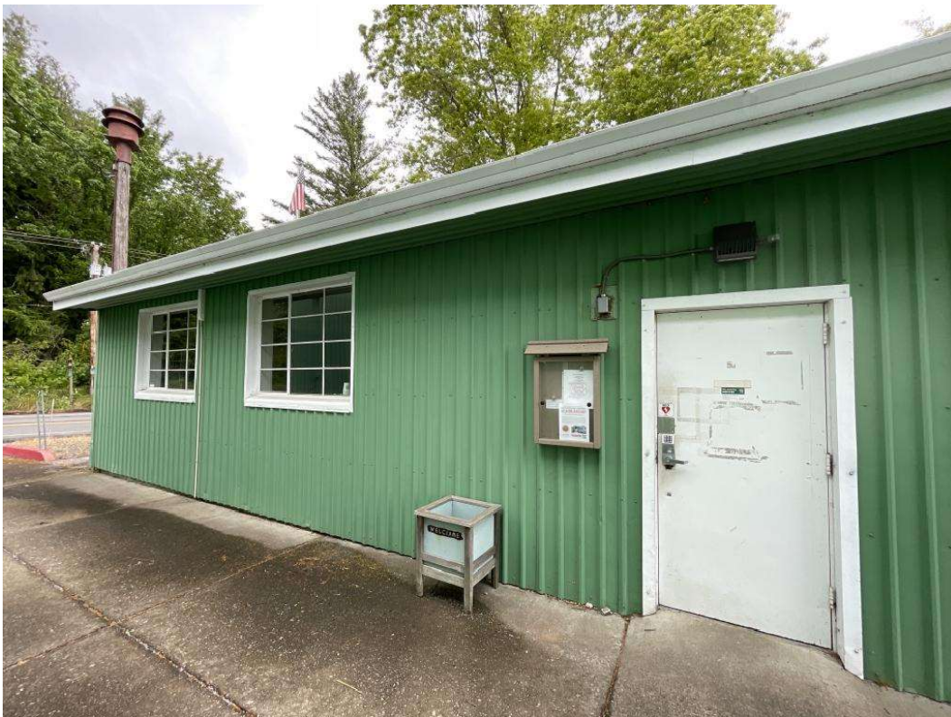
Figure 9: West elevation of the Corbett Fire Hall. View 42°. Photo Taken 05/12/2025.
