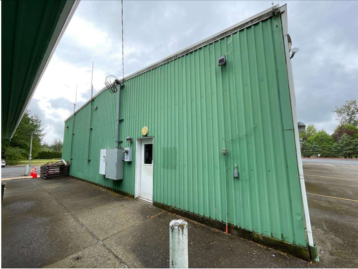
Figure 6: East elevation of the Corbett Fire Station. View 200°. Photo taken on 05/12/2025
