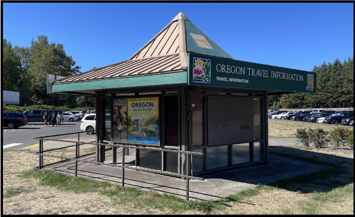
Figure 4: Rear (east) elevation of the information Kiosk. View 266°. Photo taken on 09/22/2025.
