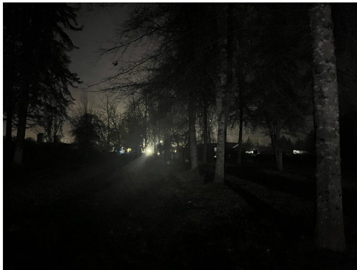
Figure 4. Lights shining from the raw water portal location on the Bull Run Filtration site immediately adjacent to residential property. Photo taken March 2, 2026 prior to approved construction hours at approximately 06:00 am
