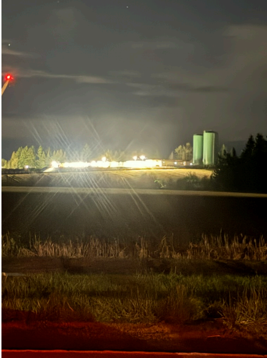
Figure 6. Photograph from SE Bluff Rd looking north, taken at approximately 7:37 p.m (March 7, 2026). Red arrows show the extent of the construction trailers at the filtration site directly west of the Pleasant Home Water District water towers.
