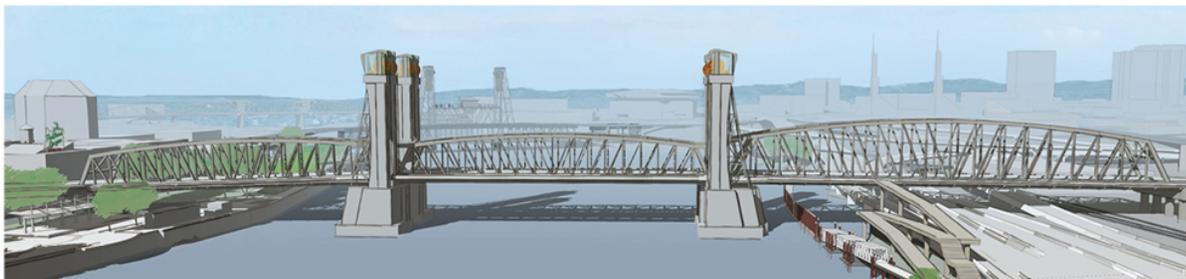
*Replacement Long Span – Through Truss Concept*
