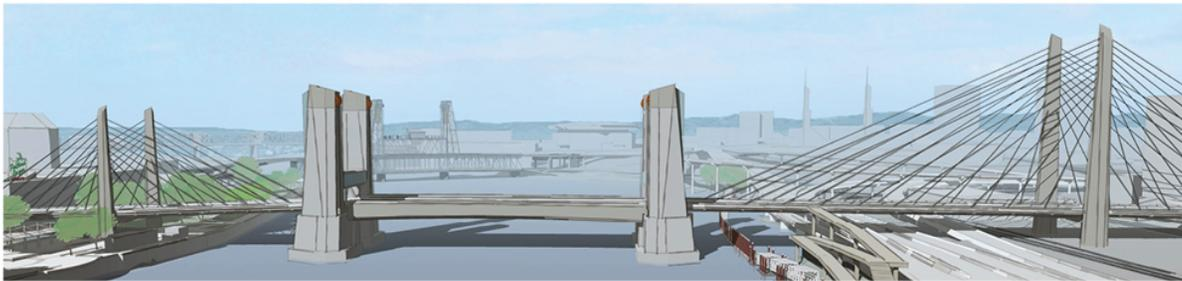
*Replacement Long Span – Cable Stayed Concept*
