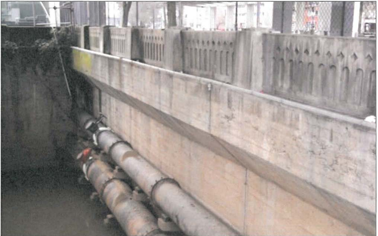
View: The Harbor Wall's original concrete bulkhead and railing where it faces Pier 1, view towards southwest.
