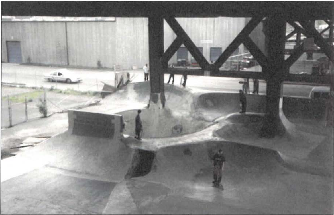
View: A view showing how the Burnside Bridge's columns have been incorporated into skating features. Looking southwest (Photo courtesy www.burnsideproject.org , used with permission).
