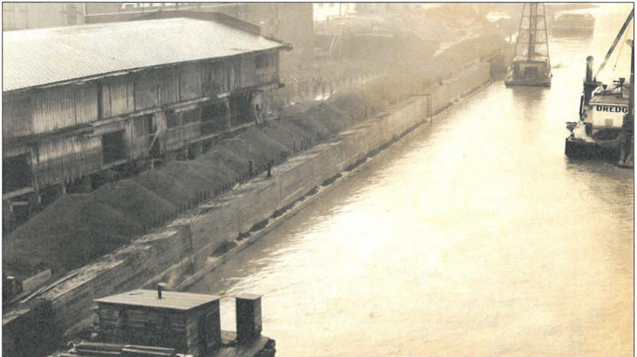
View: Portland Harbor Wall under construction in 1928, view facing northwest.
