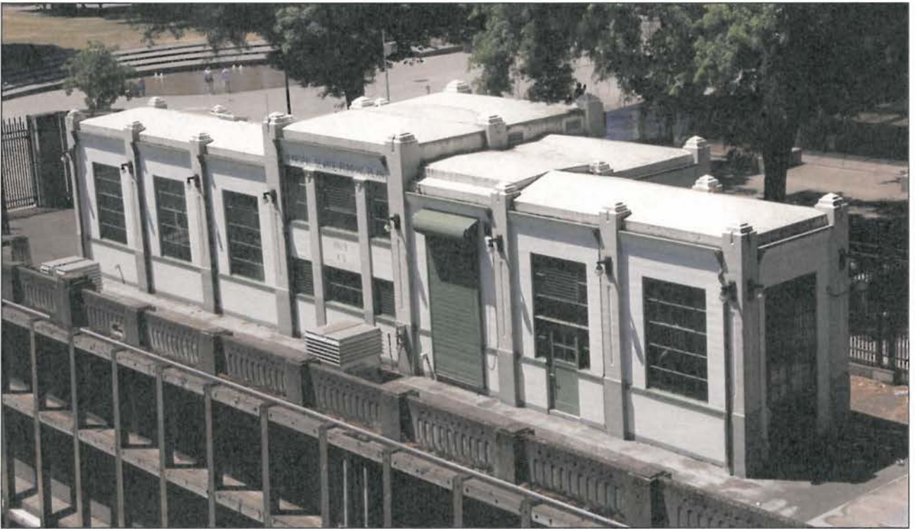
View: The east and north facades of the Ankeny Pumping Station; the view is towards the southwest.
