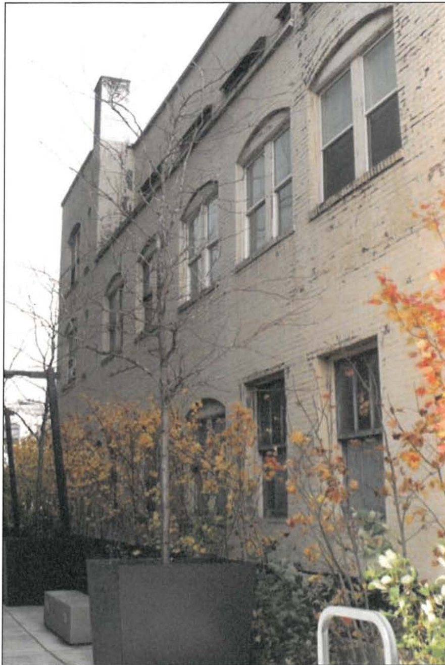
View: The north and west facades showing the differences from the detailed north façade and the utilitarian west façade. The view is towards the southeast.
