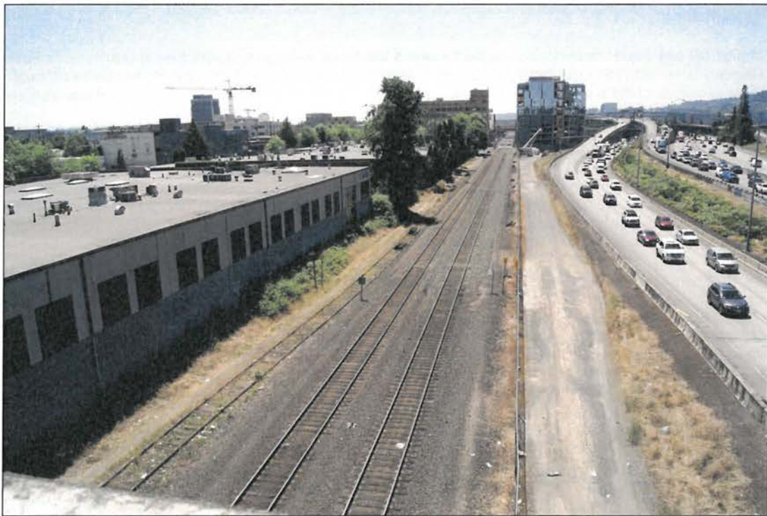
A view of the historic alignment of the Oregon and California RR where it travels along SE First Avenue. The view is towards the south with Interstate 5 to the right.
