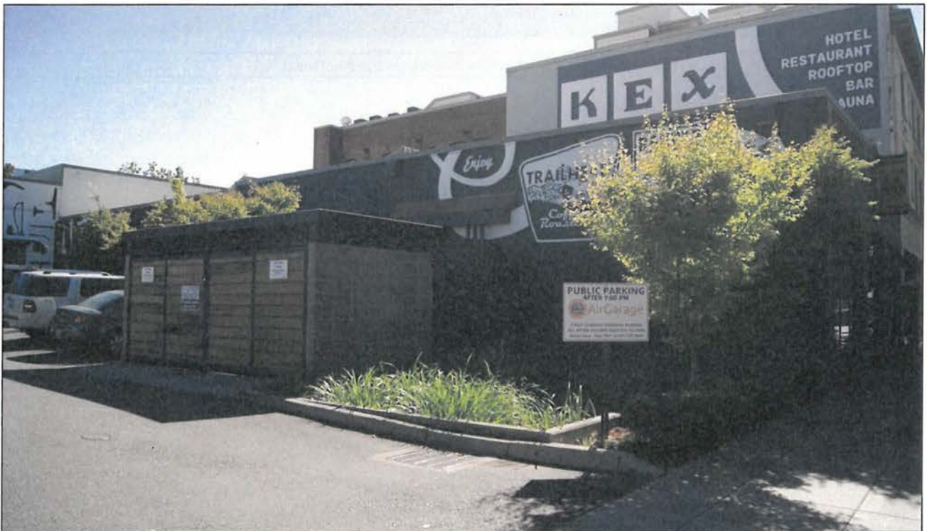
View: A view of the building's north façade; the view is towards the southeast.
