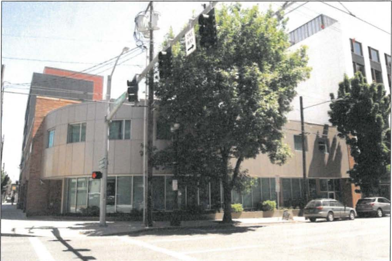
View.: The west building segment's west façade; the view is towards the southeast.
