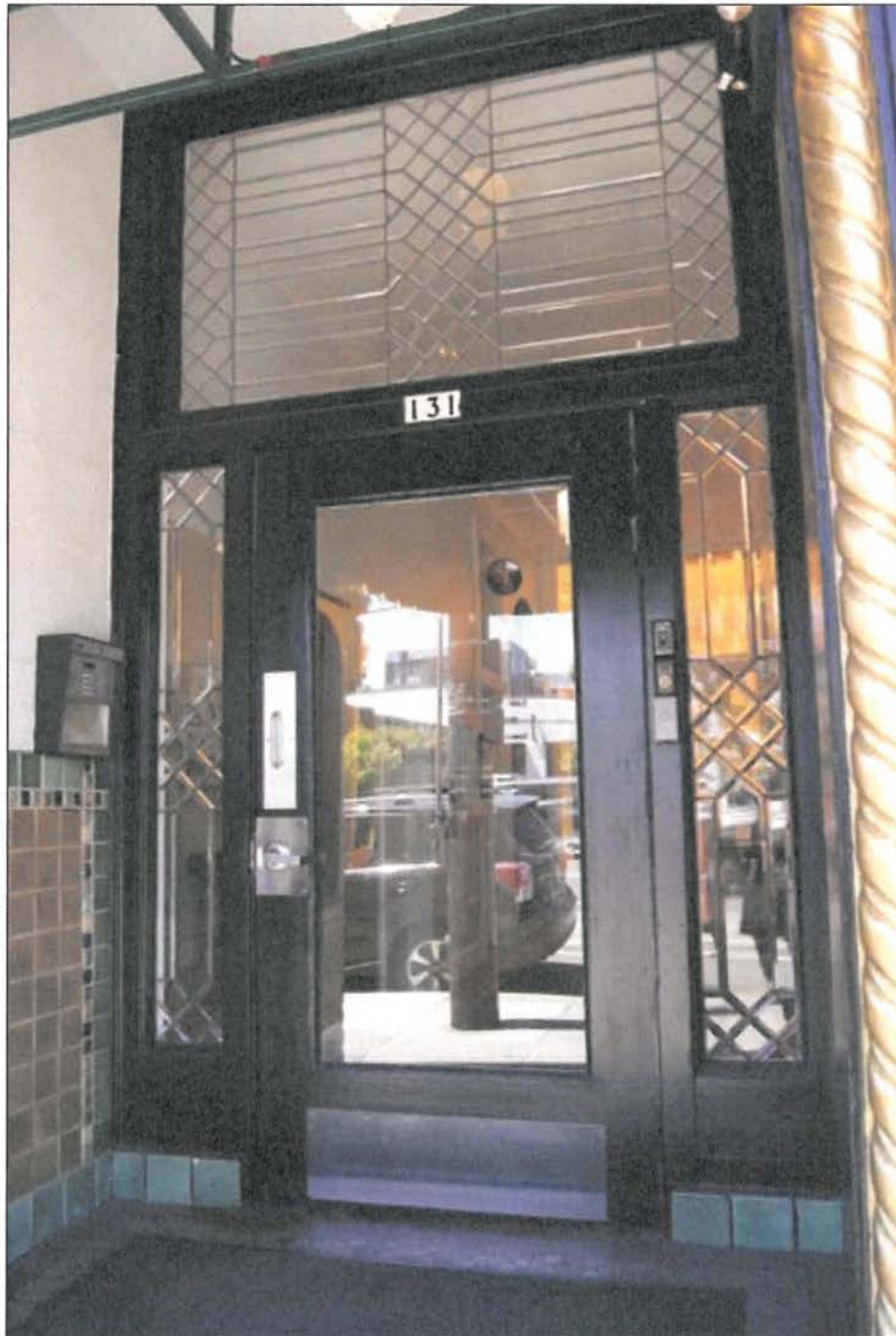
View: A detail of the main entry on the east façade showing the cable surround, colorful tile, and leaded glass sidelights and transom. The view is towards the west.
