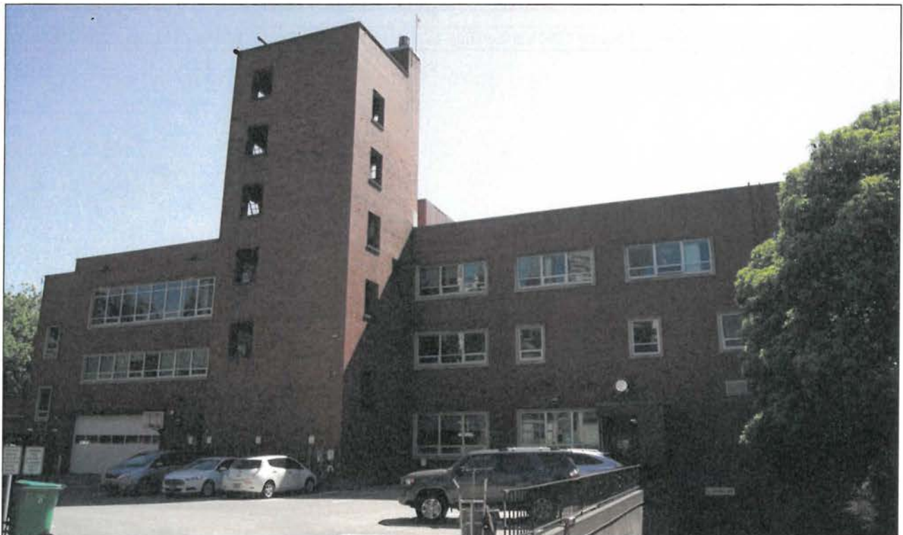
View: The rear (west) façade of the Central Fire Station. The view is towards the northeast.
