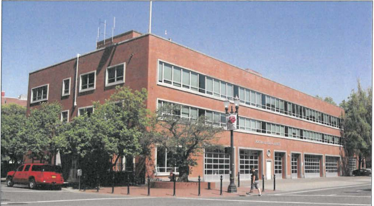
View: Central Fire Station's south and east facades. The view is towards the northwest.
