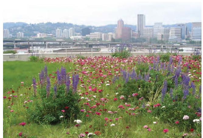
Multnomah Building Green Roof
