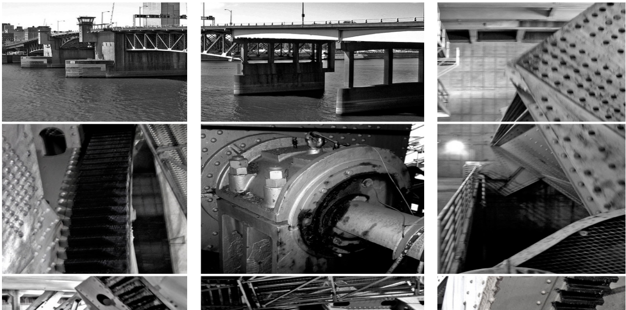
Photo Credit: Morrison Bridge by Jeff Kubina
