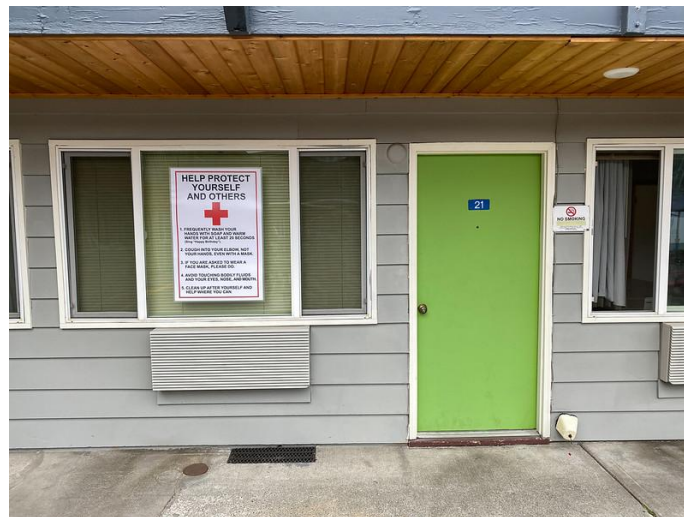
Shelter opening at the Banfield Value Inn for people to self-isolate and recover from Covid-19.
