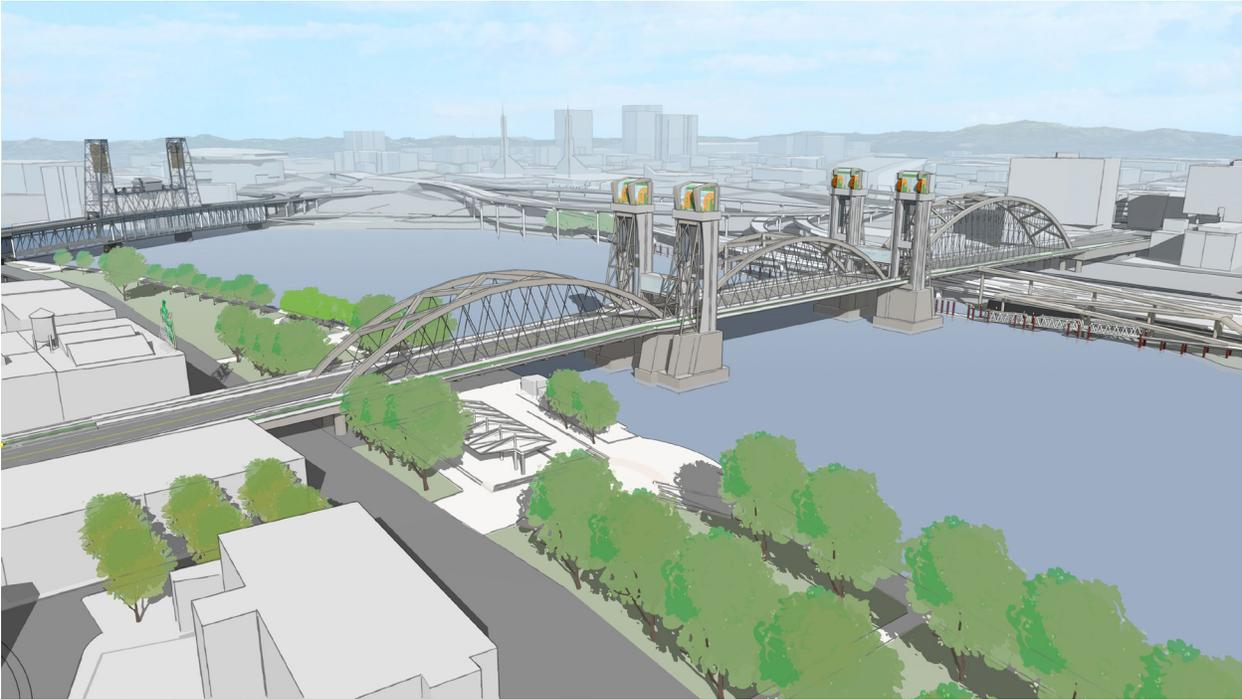
Figure 12. Long-Span Alternative: Bascule Lift Option and Cable-Stayed Configuration
