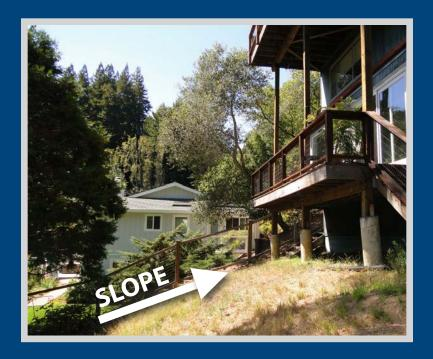
Managing vegetation on the slope is important for reducing the exposure to the deck and minimizing the chance of ignition from a wildfire. Fire burning up the slope to the deck can expose the bottom and top of the deck to heat, flames and embers.
