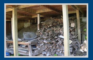
No deck, regardless of the material used to build it, would be safe if this amount of fuel beneath the deck caught fire. Even decks that may have a noncombustible surface, such as light-weight concrete, use lumber and timbers for structural support and those materials can catch fire.
