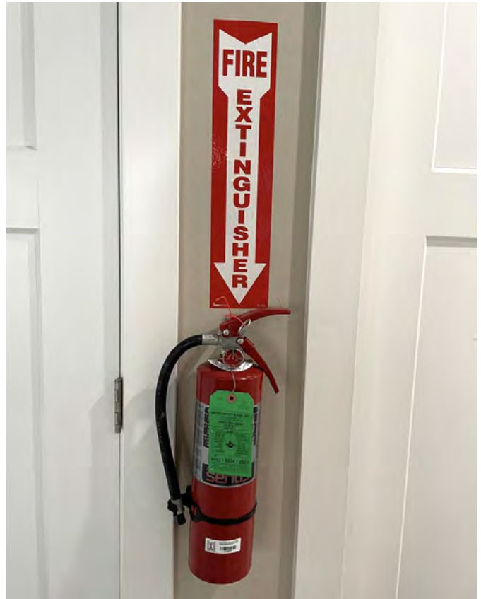
Mounted fire extinguisher between bedroom doors.
