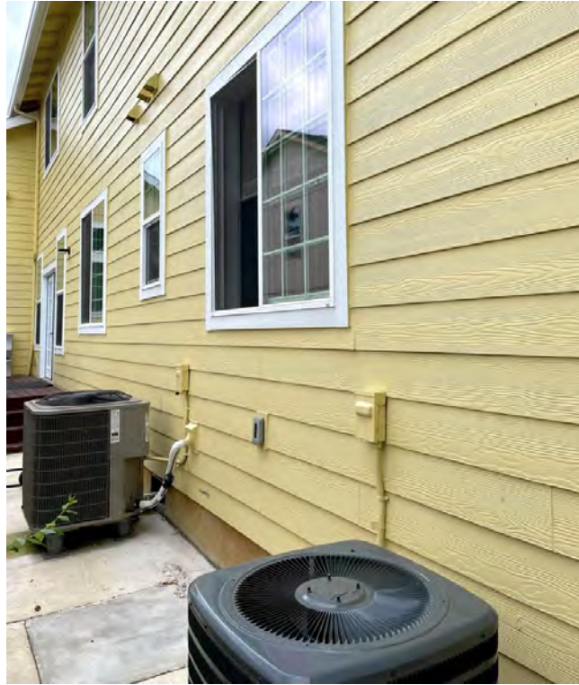
Air conditioner units do not block the resident's window, which is the secondary exit.
