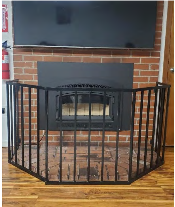
Custom-made barrier for fireplace or wood stove, with fire extinguisher located nearby.
