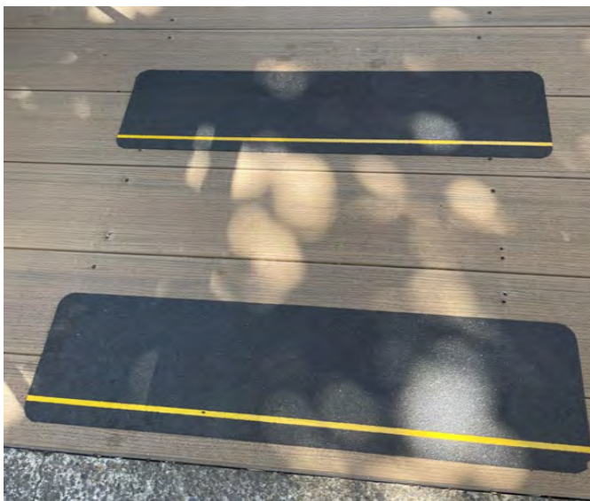
Additional slip resistance added to the floor.
