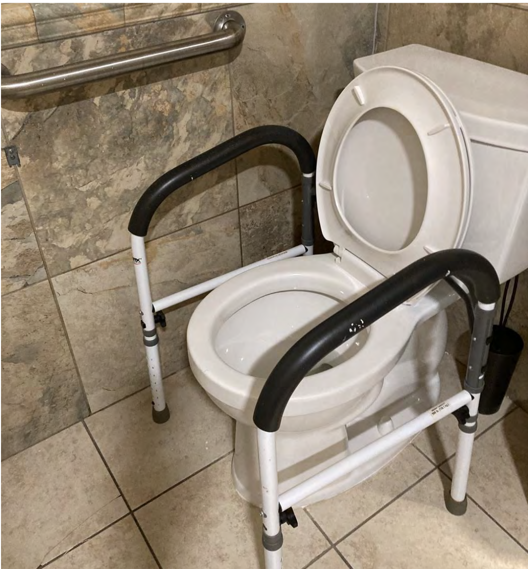
Grab bars on wall and toilet safety rail.
