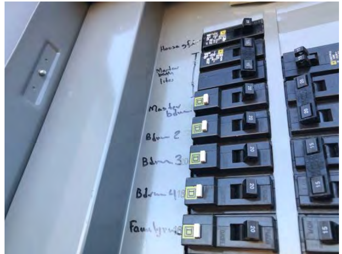
Electrical panel box with room labeling.
