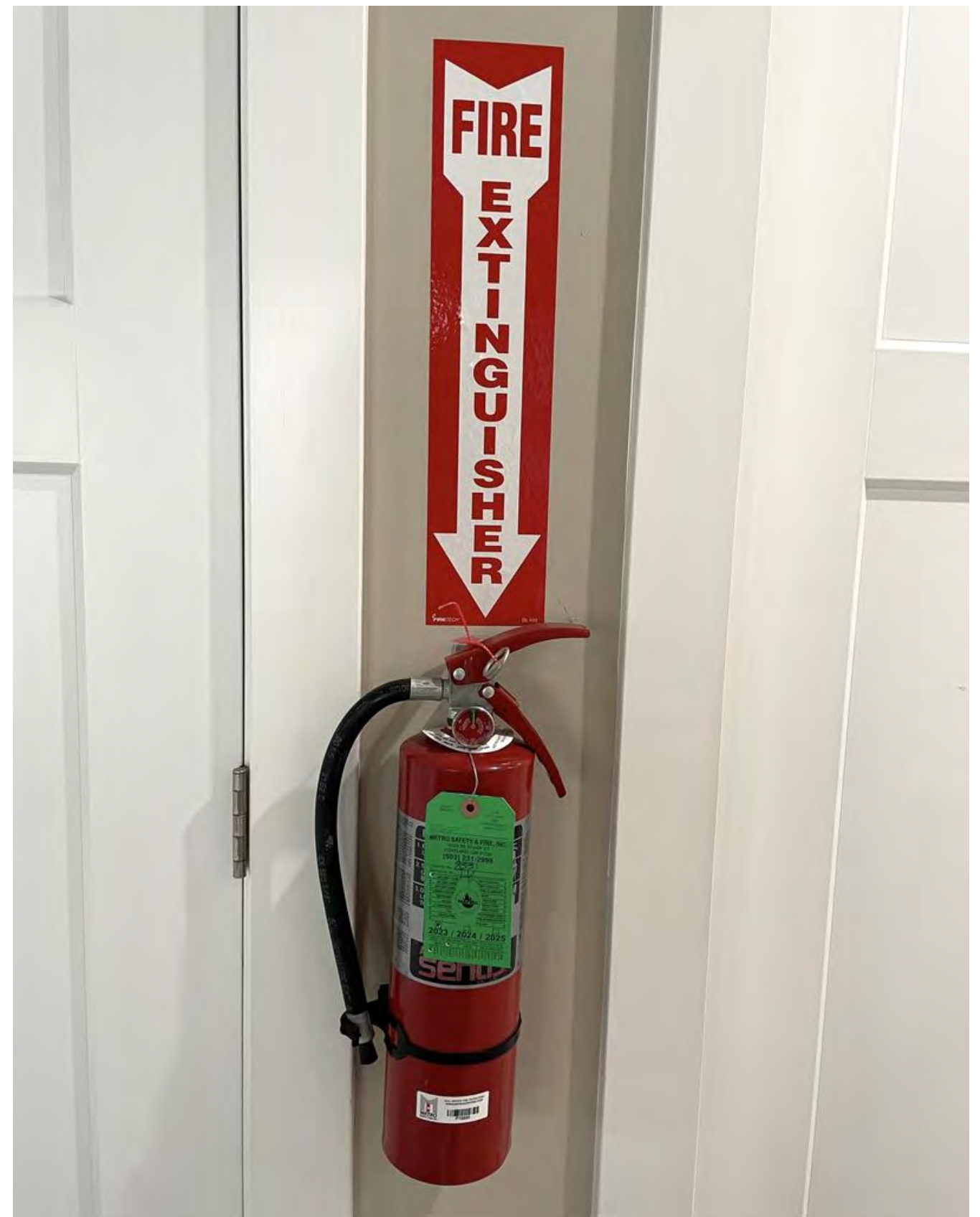
Mounted fire extinguisher between bedroom doors.
