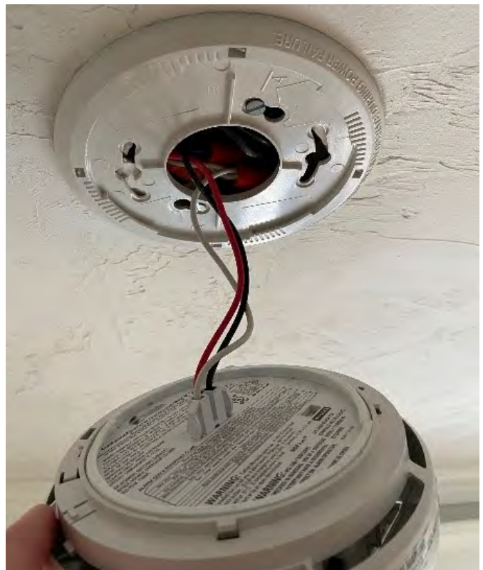
A smoke alarm hardwired into the ceiling.
