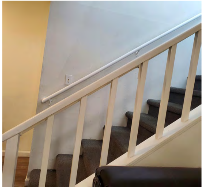
Guardrail with vertical pattern.
