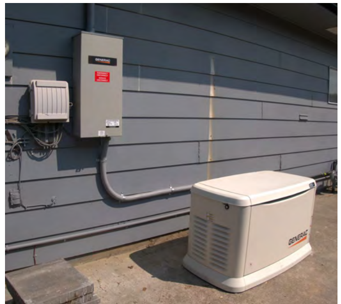
Generator connection.
