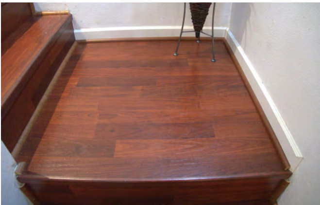
Stairway landing between two flights of stairs, equal to the width of the stairs.
