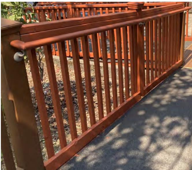
Edge protection barrier from guardrails to ramp floor. Edge protection is flush to the ground, meeting the ADA requirements.
