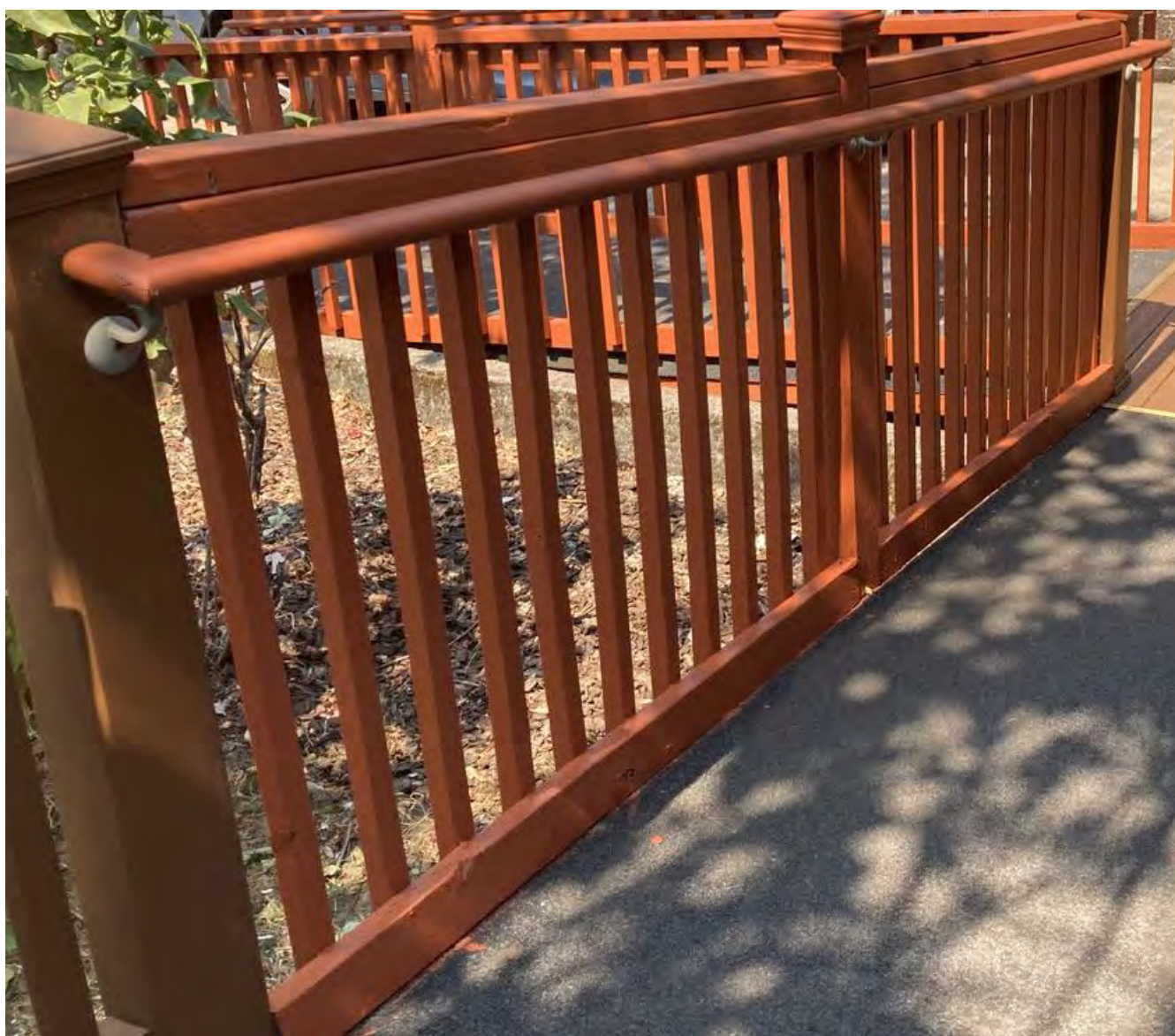
Edge protection barrier from guardrails to ramp floor. Edge protection is flush to the ground, meeting the ADA requirements.
