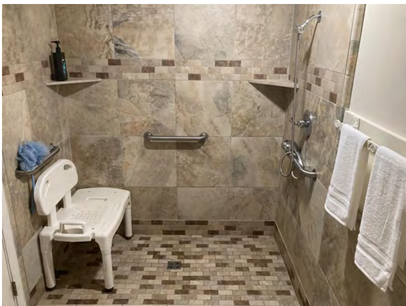
Accessible shower with foldable shower seat and grab bar.
