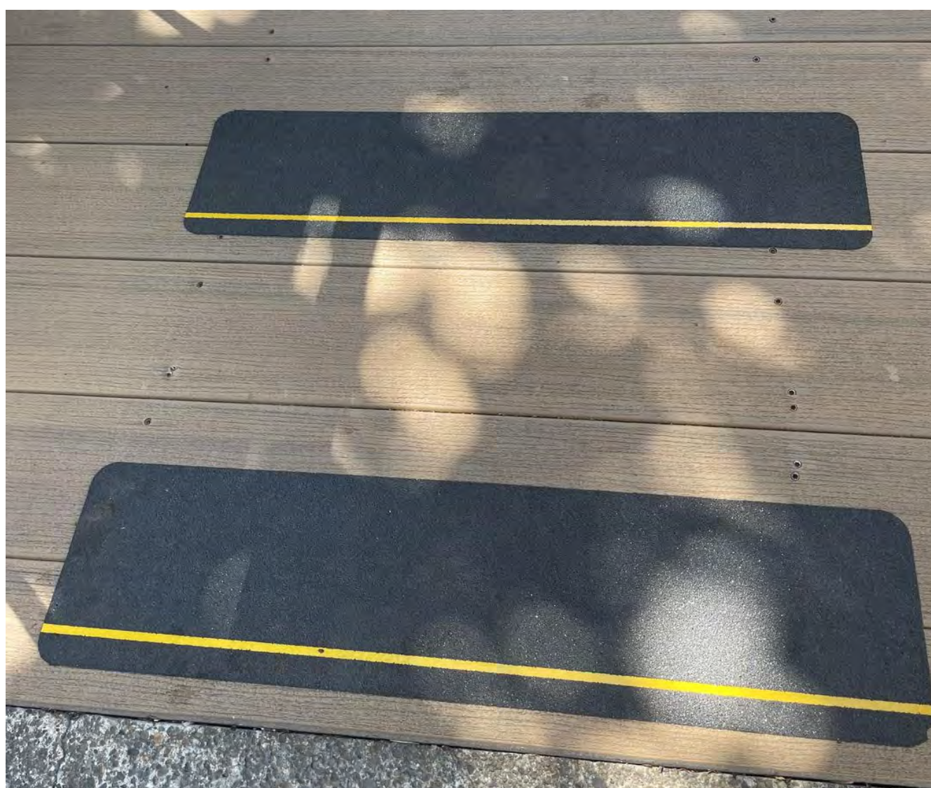
Additional slip resistance added to the floor.
