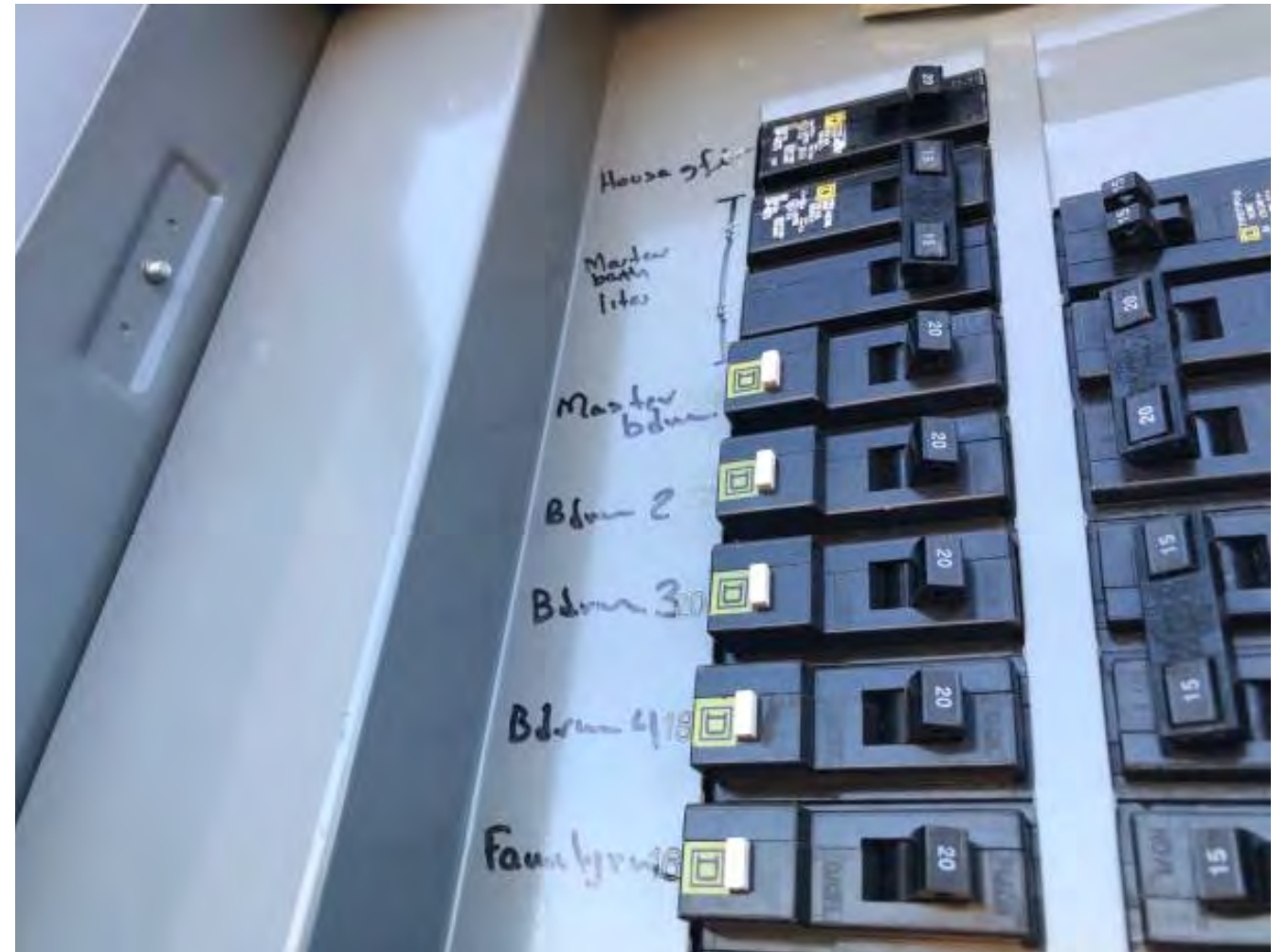
Electrical panel box with room labeling.
