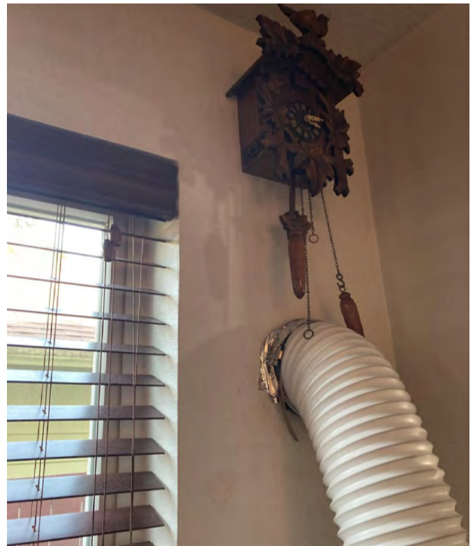
Portable air conditioner with hose going through wall does not block window.
