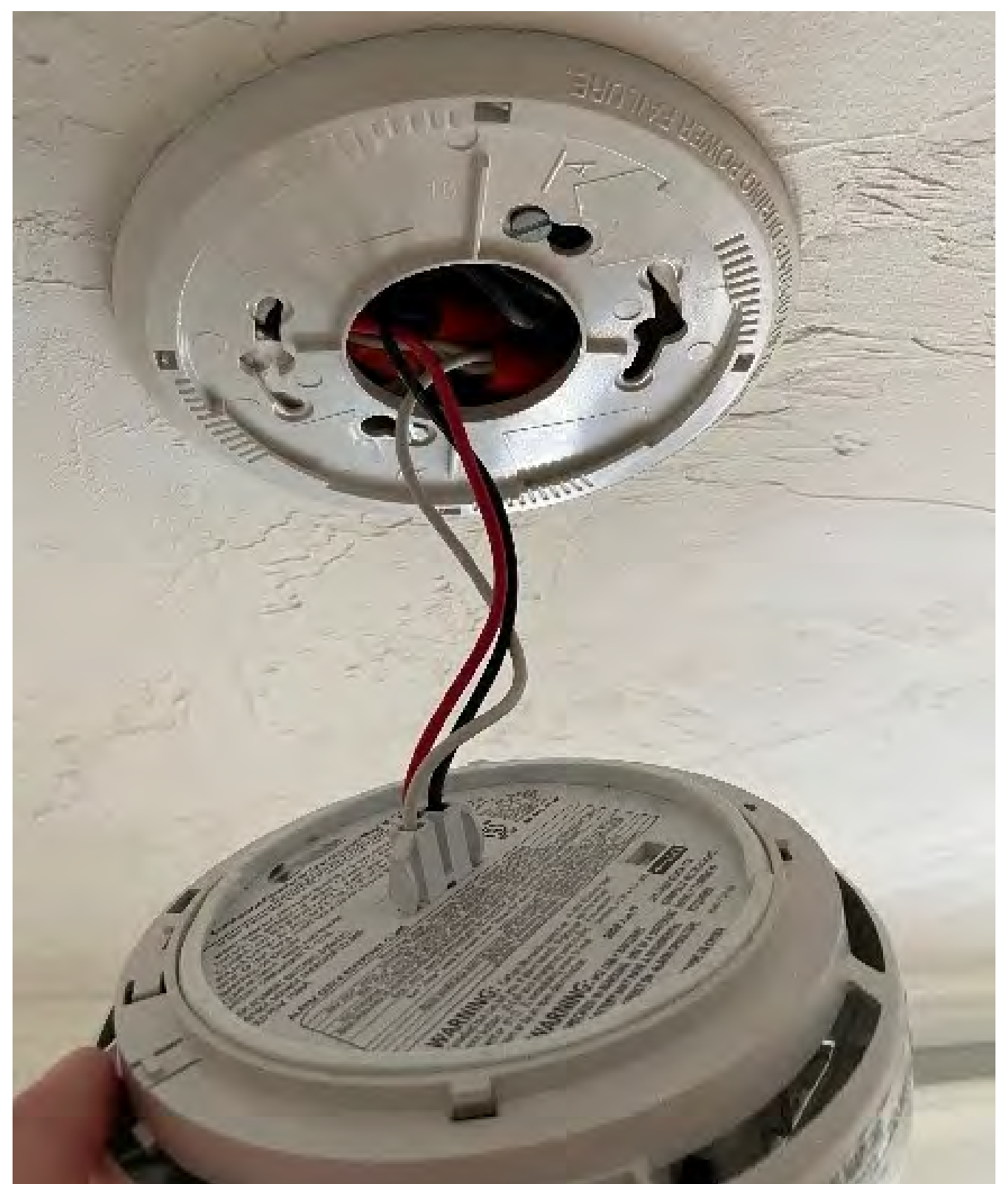
A smoke alarm hardwired into the ceiling.
