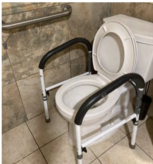
Grab bars on wall and toilet safety rail.
