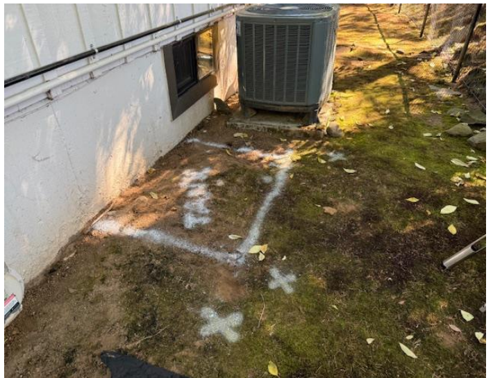
8. Marked former heating oil tank (HOT) location, adjacent to southern elevation of single family residence
