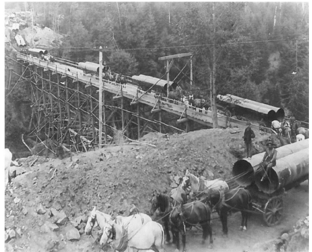
Figure 2. Pipeline Construction in the late 1800s
