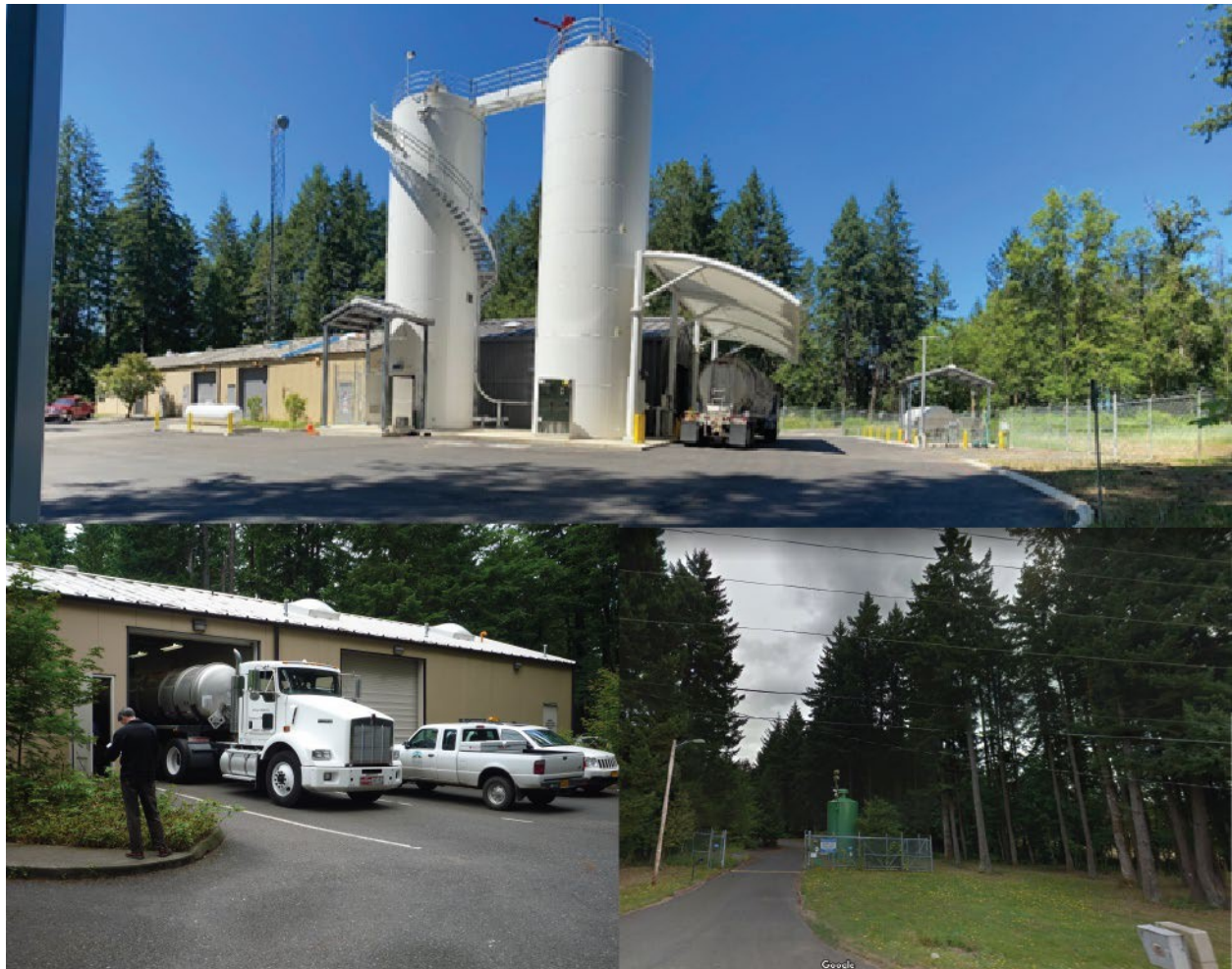
Figure 13. Lusted Hill Treatment Facility (6704 Cottrell Road #10)
