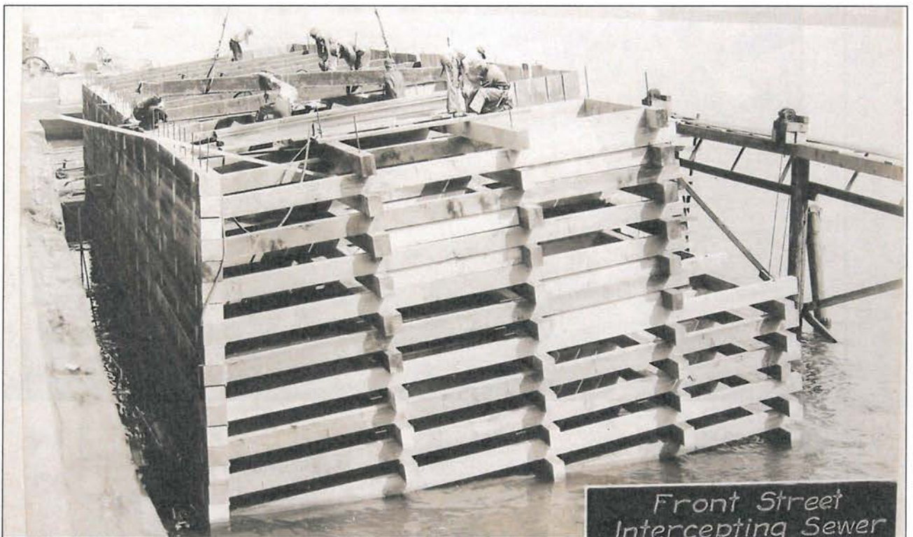
View: A typical cross section of Portland Harbor Wall cribbing from Olaf Laugaard's (1933) treatise.
