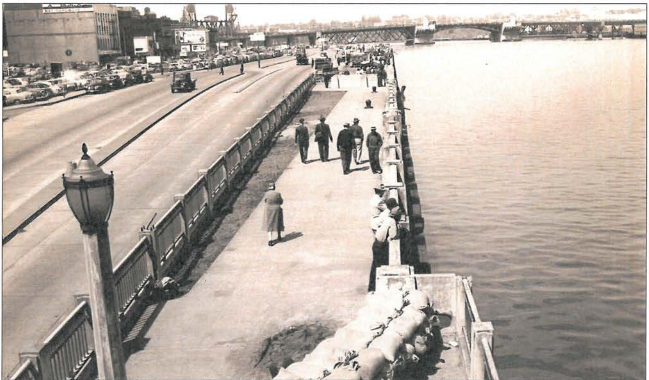
View: Portland Harbor Wall prepared for the 1948 Flood. Burnside Bridge is viewed to the north.
