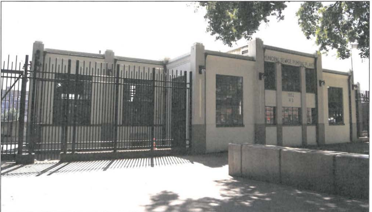
View: The Ankeny Pumping Station's east façade; the view is towards the southeast.
