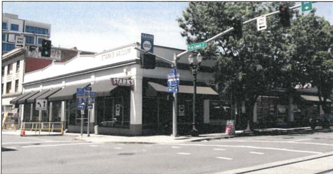
Stark's Vacuum Company's south building segment showing the south and east facades; view to the northwest.
