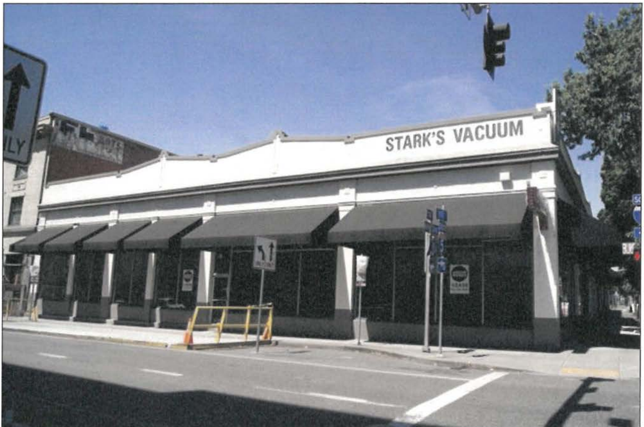
View: The south building segment (1926) showing the south façade; the view is to the north-northwest.
