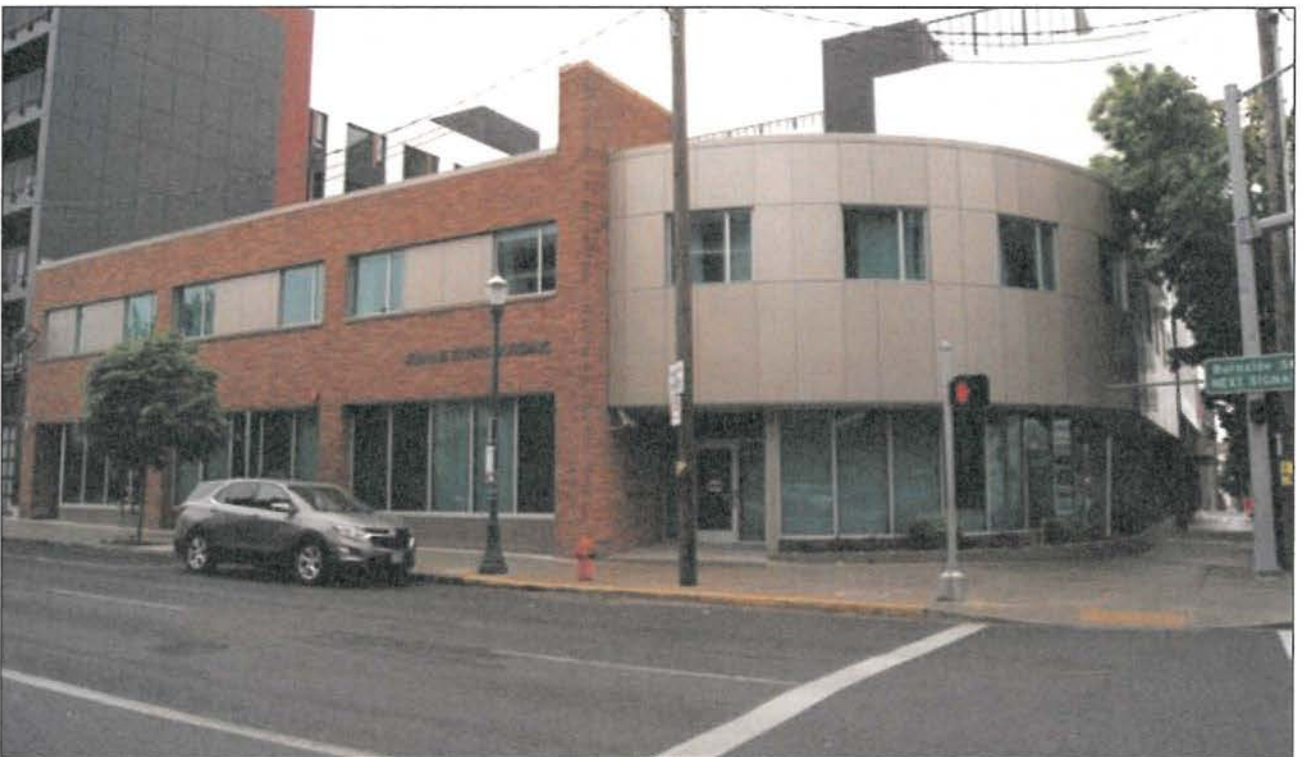
View: A closer view of the transition between the east and west building segments; the view is to the southeast.
