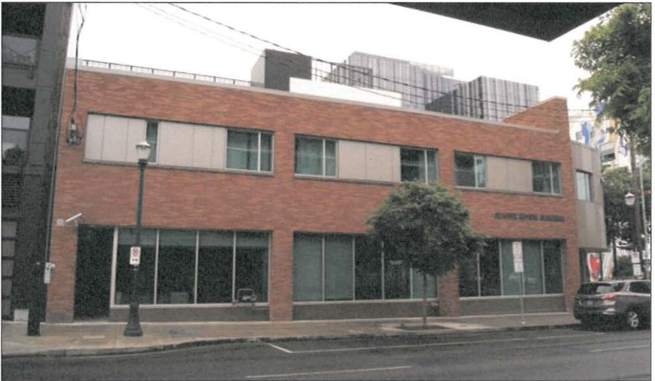
View: The north façade of 30 NE Martin Luther King Blvd. Building looking southwest.
