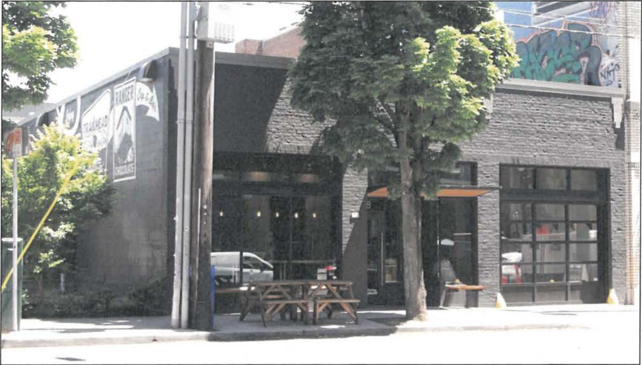
View: A view of the building's west façade; the view is towards the east.
