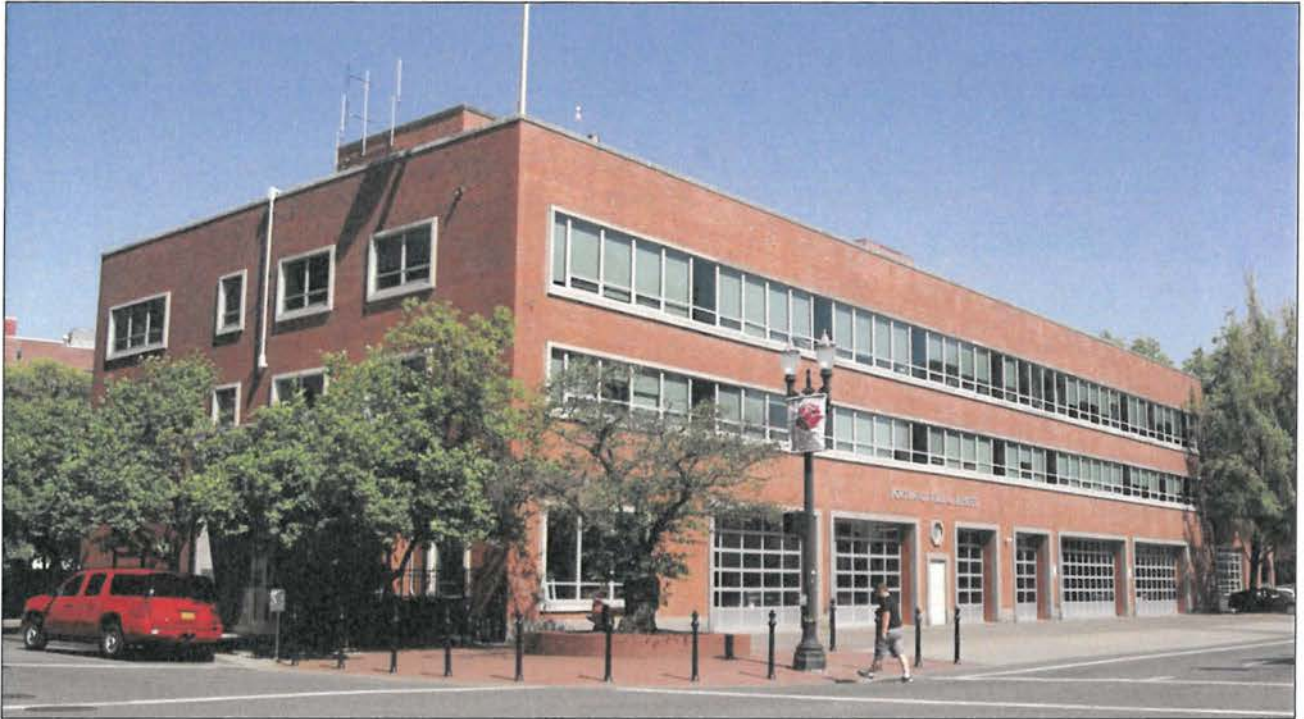
View: Central Fire Station's south and east facades. The view is towards the northwest.
