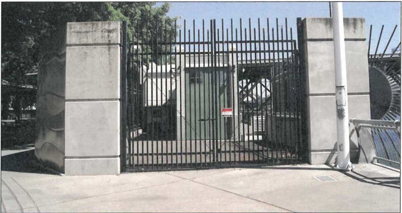
View: The south façade of the Ankeny Pumping Station; the view is towards the north.
