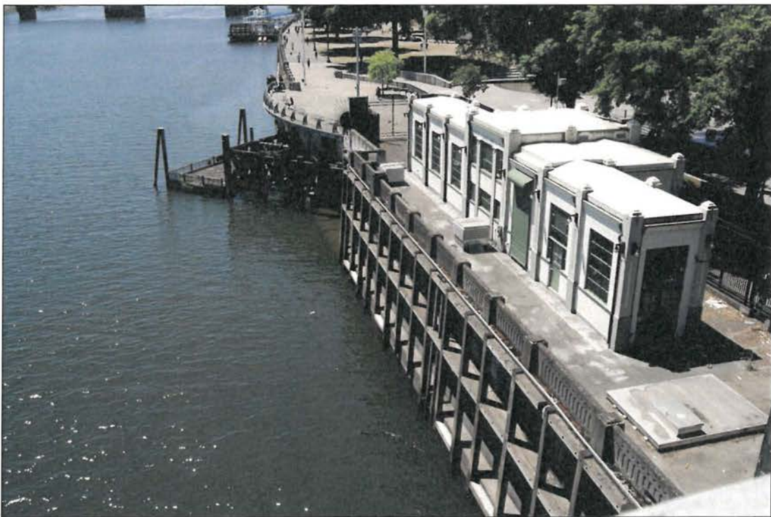
A view of the Portland Harbor Wall and the Ankeny Pumping Station taken from the Burnside Bridge; the view is towards the southwest. Note the original concrete rail panels adjacent to the pumping station.
