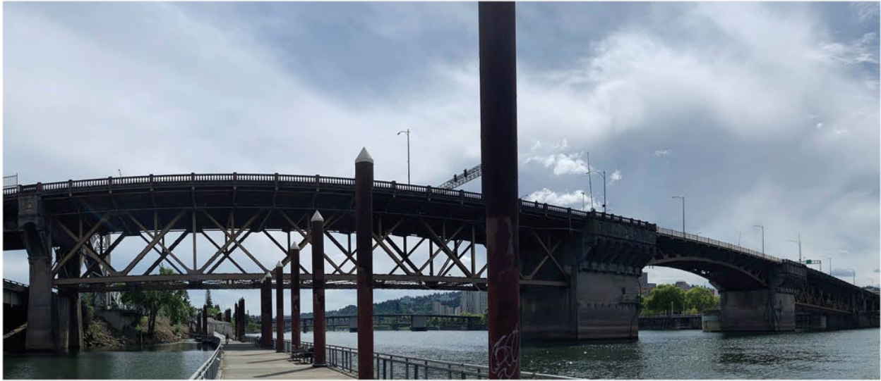
Figure 2-2. View of the Vera Katz Eastbank Esplanade, Looking South under the Burnside Bridge
