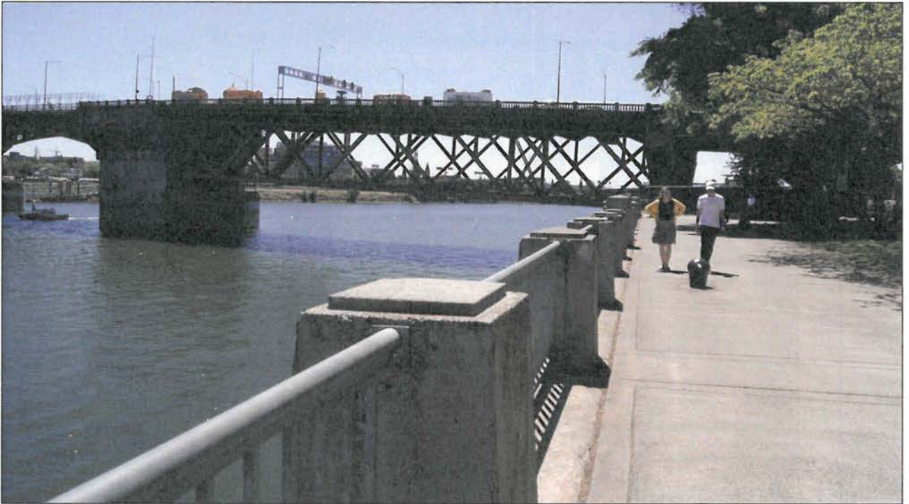
View: Portland Harbor Wall and an example of the 1977 railing modification; the view is towards south.
