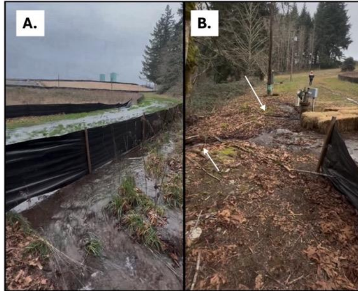
Figure 12. Overland flow of groundwater pumped from the filtration construction site and directed into Johnson Creek. ( Photo credit: Jennifer Hart; January 30, 2025 ). (A) Approximately 1,600 gallons per minute, or 3-4 cfs, is being pumped into Johnson Creek on workdays (6 days per week), 10-11 hours per day, suddenly increasing and decreasing stream flow on a regular basis. (B) Excessive discharge of significant volumes of water creates channelization and sediment transport into Johnson Creek ( see white arrows ) negatively impacting the riparian habitat and the naturally occurring water quality conditions of the creek.
