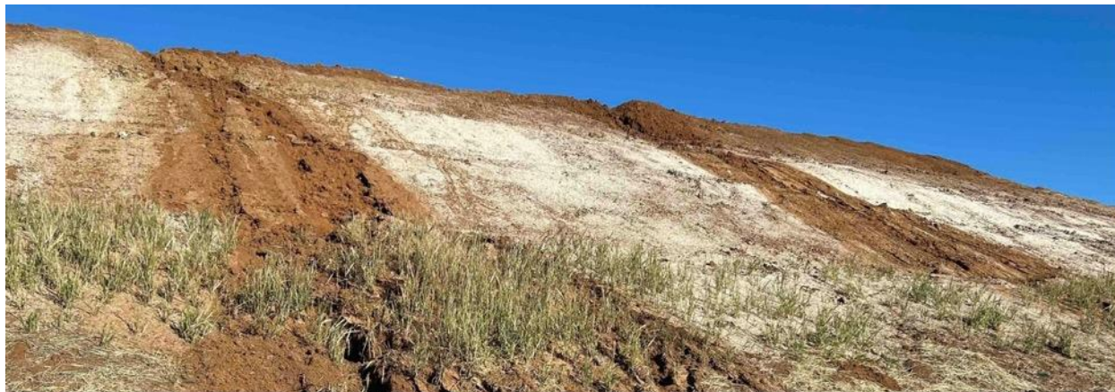
Figure 14. Example of erosion occurring at PWB's construction site.
