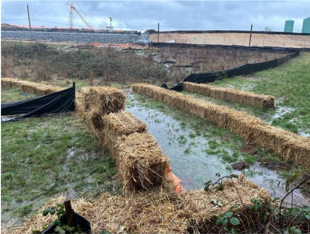
Figure 5. Stormwater discharge from PWB’s construction site directed into Johnson Creek and its associated riparian area through the use of hay bales and silt fencing (February 2025). Hay bales were installed as a form of erosion control after formal complaint made by community members to Oregon Water Resources Department and the Oregon Department of Environmental Quality in January 2025. Hay bales did not alleviate erosion, channelization, or increased sedimentation of Johnson Creek.
