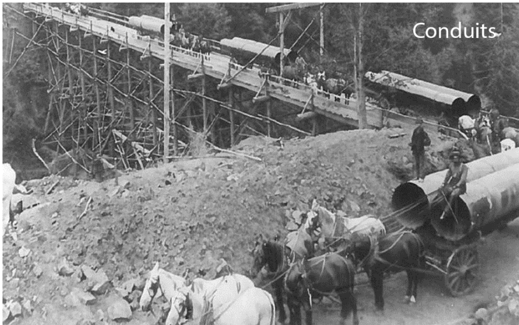
Pipeline construction in late 1800s.
