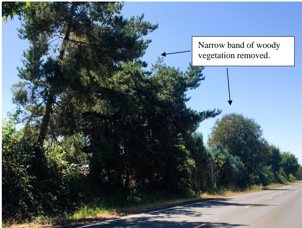
Photograph 6. A single row of shrubs/trees on the south side of SE Dodge Park Boulevard removed during construction (August 2023).
