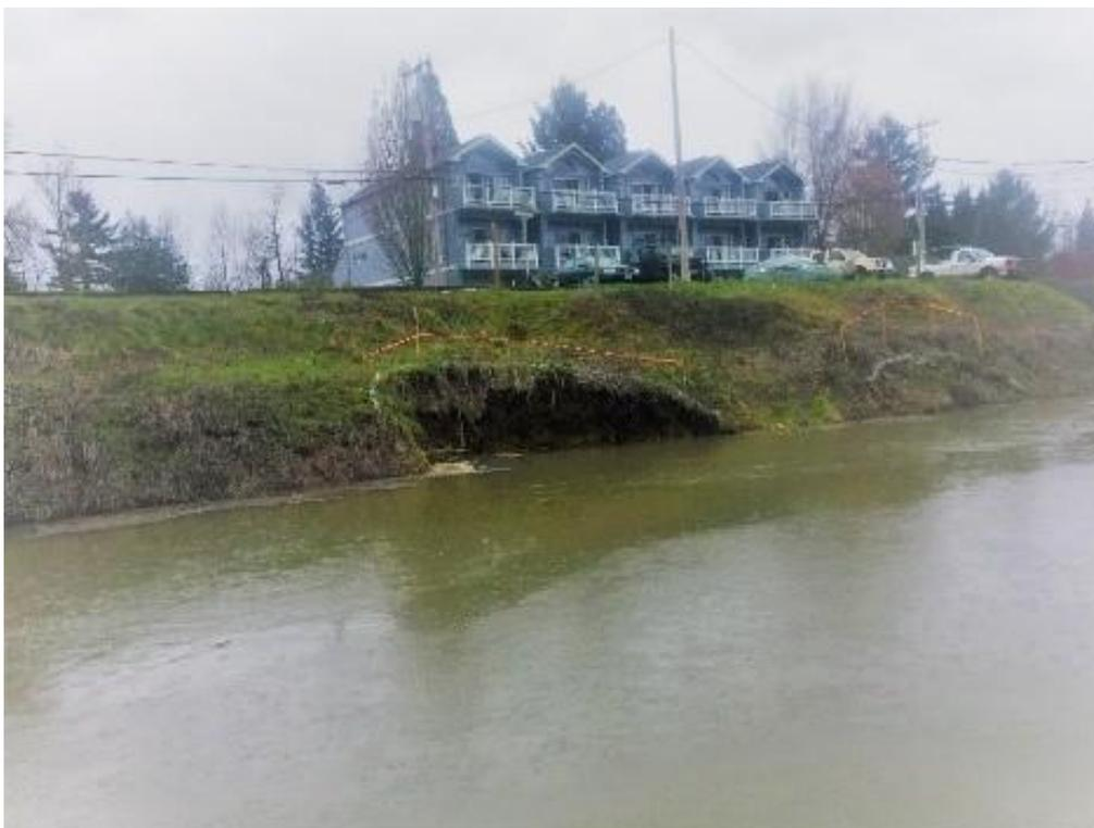
*Figure 46 - Levee sloughing damage near NE Bridgeton Rd., in Portland caused by high water during the Spring 2017 flood event. Photo Multnomah County Drainage District.*
