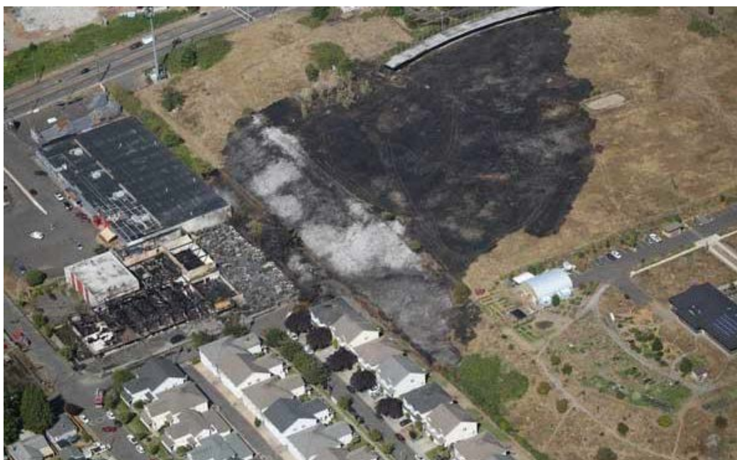
Figure 97 - Aerial photo of damage from the 2019 fire in Portland. Photo Portland Fire
