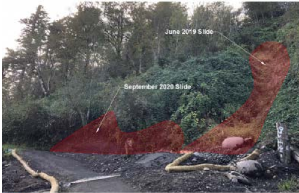
Figure 139 - Map showing location on landslides on Robin's Way Trail in 2019 and 2020. Graphic - City of Troutdale
