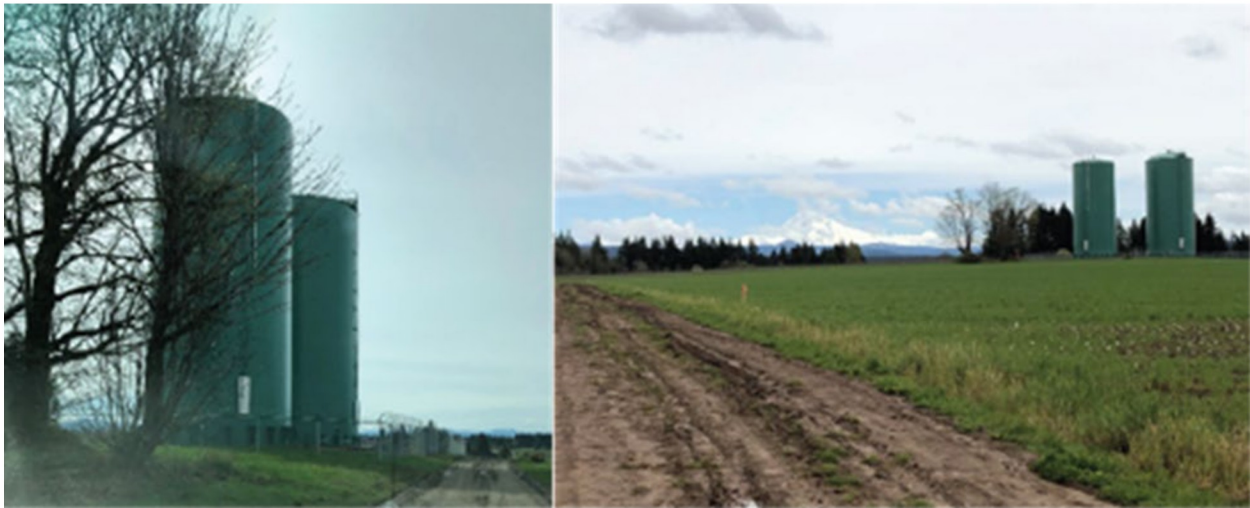
Figure 15. PHWD Water Tanks (35524 Carpenter Lane #9)
