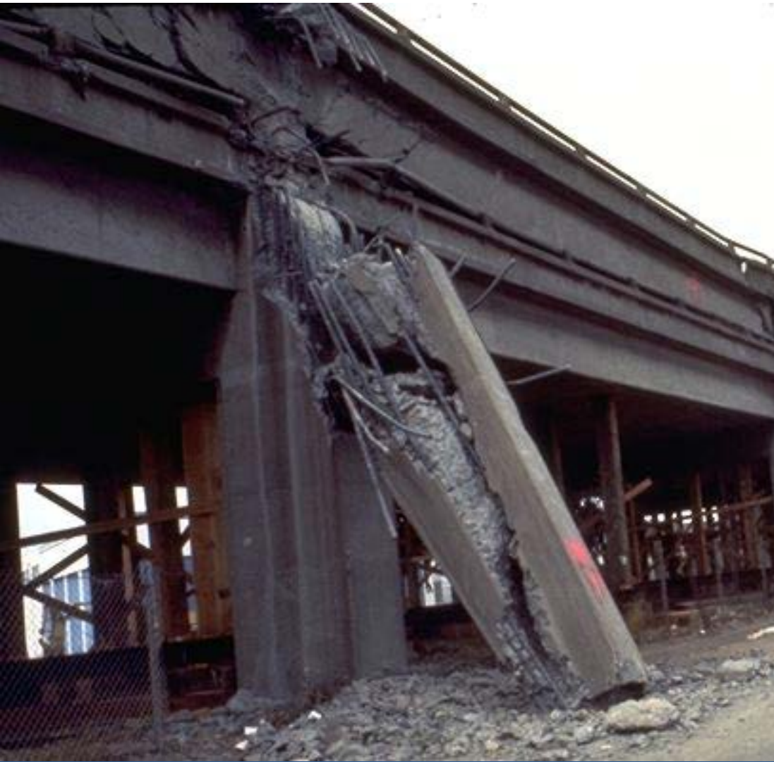
1989 Loma Prieta Earthquake Column Failure
