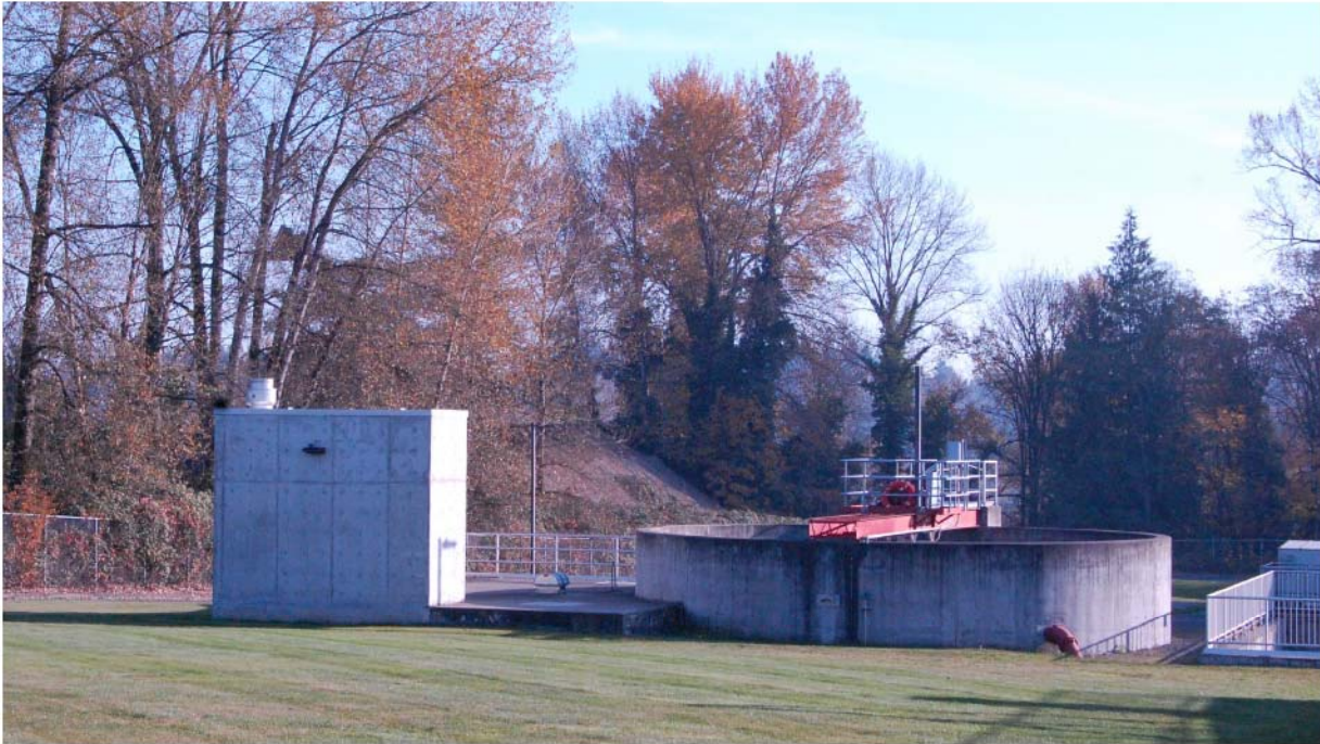
Figure 2. Below grade sludge equalization storage (left) seen during the Wilsonville Water Treatment Plant tour.
