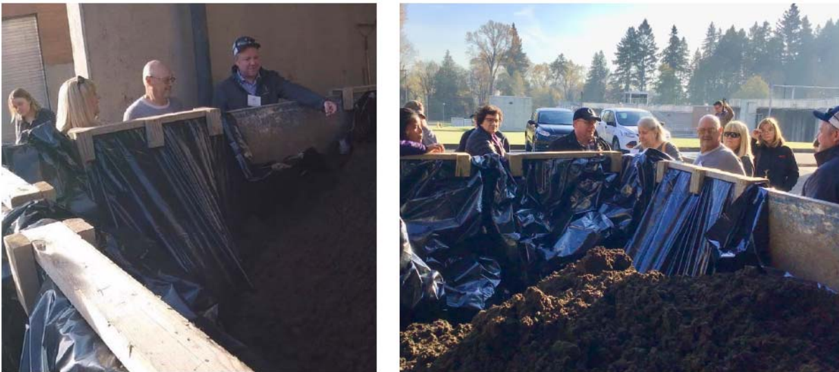
Figure 3. Typical residual solids seen in a roll-off bin near the chemical building during the Wilsonville Water Treatment Plant tour.
