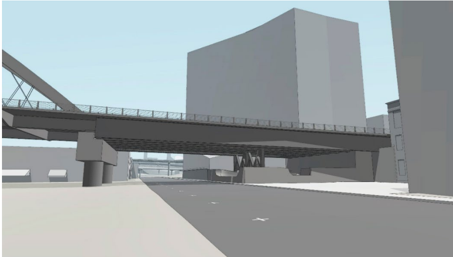
Figure 16. View of East Pier, Refined Long-Span, Tied-Arch, West Side of 2nd Avenue
