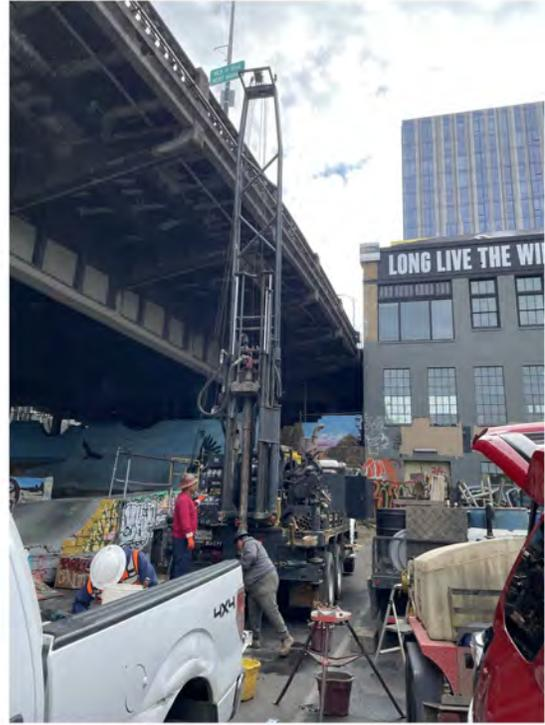
**Photo 14** - View of drilling set up at boring B-18 adjacent to SE 2nd Ave.
