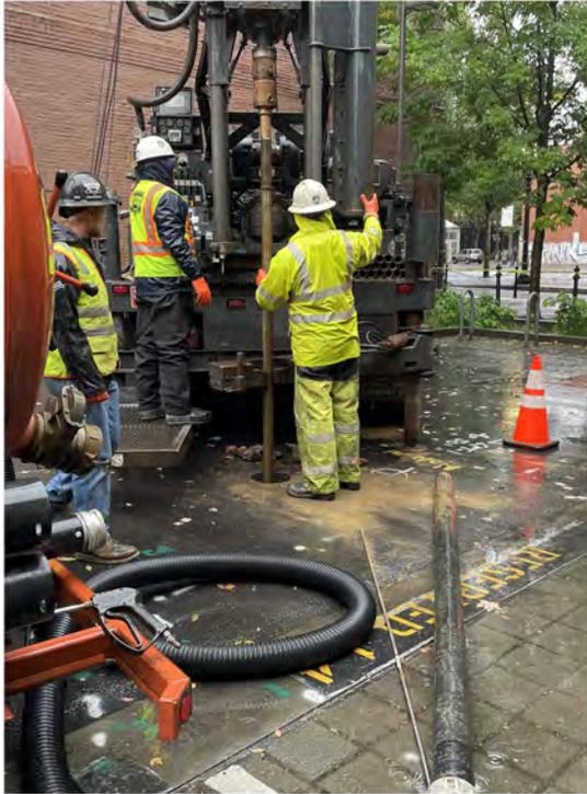
**Photo 1** - View of drilling at boring B-5 in the Mercy Corps parking lot near SW 1st Ave.
