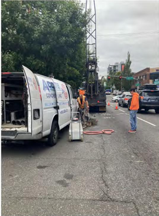
**Photo 17** - View of pavement coring for boring B-20 along E Burnside St near NE/SE Martin Luther King Jr Blvd.
