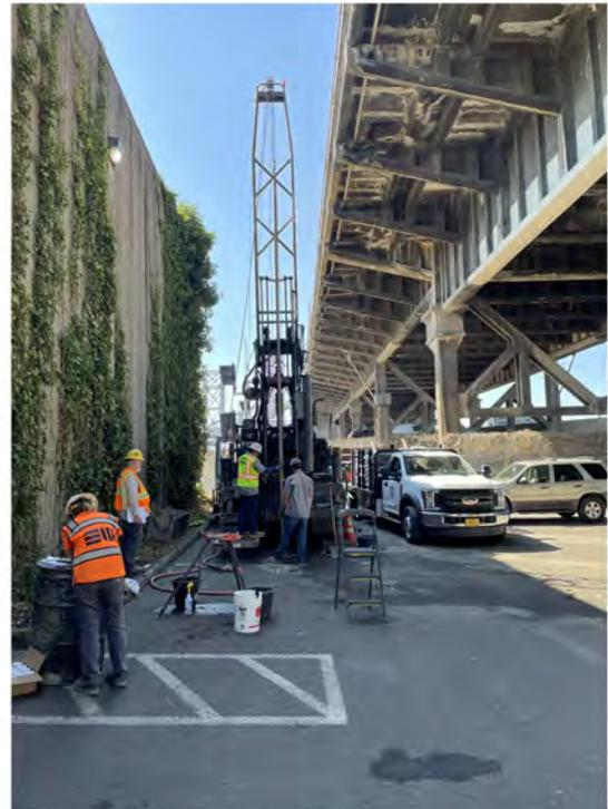
**Photo 20** - View of drilling activities at boring B-33 adjacent to the AMR maintenance building.
