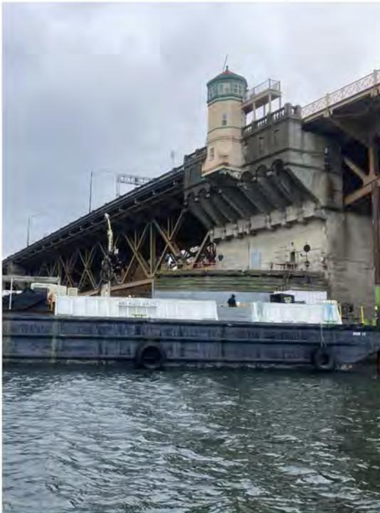
**Photo 27** - View of barge and drilling set up at in-water boring B-30, south of the bridge.
