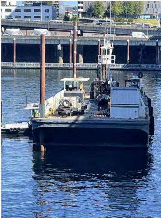
**Photo 23** - View of barge and drilling set up at in-water boring B24, north of the bridge.
