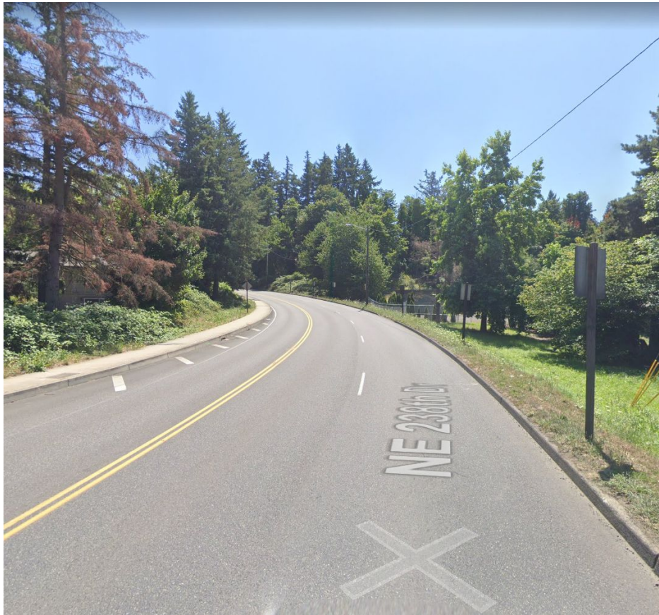
Before and After - Looking south up the hill
