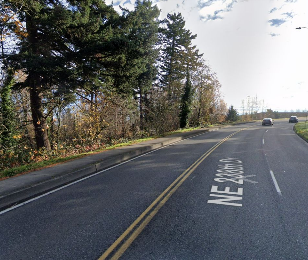
Before and After - Looking south up the hill
