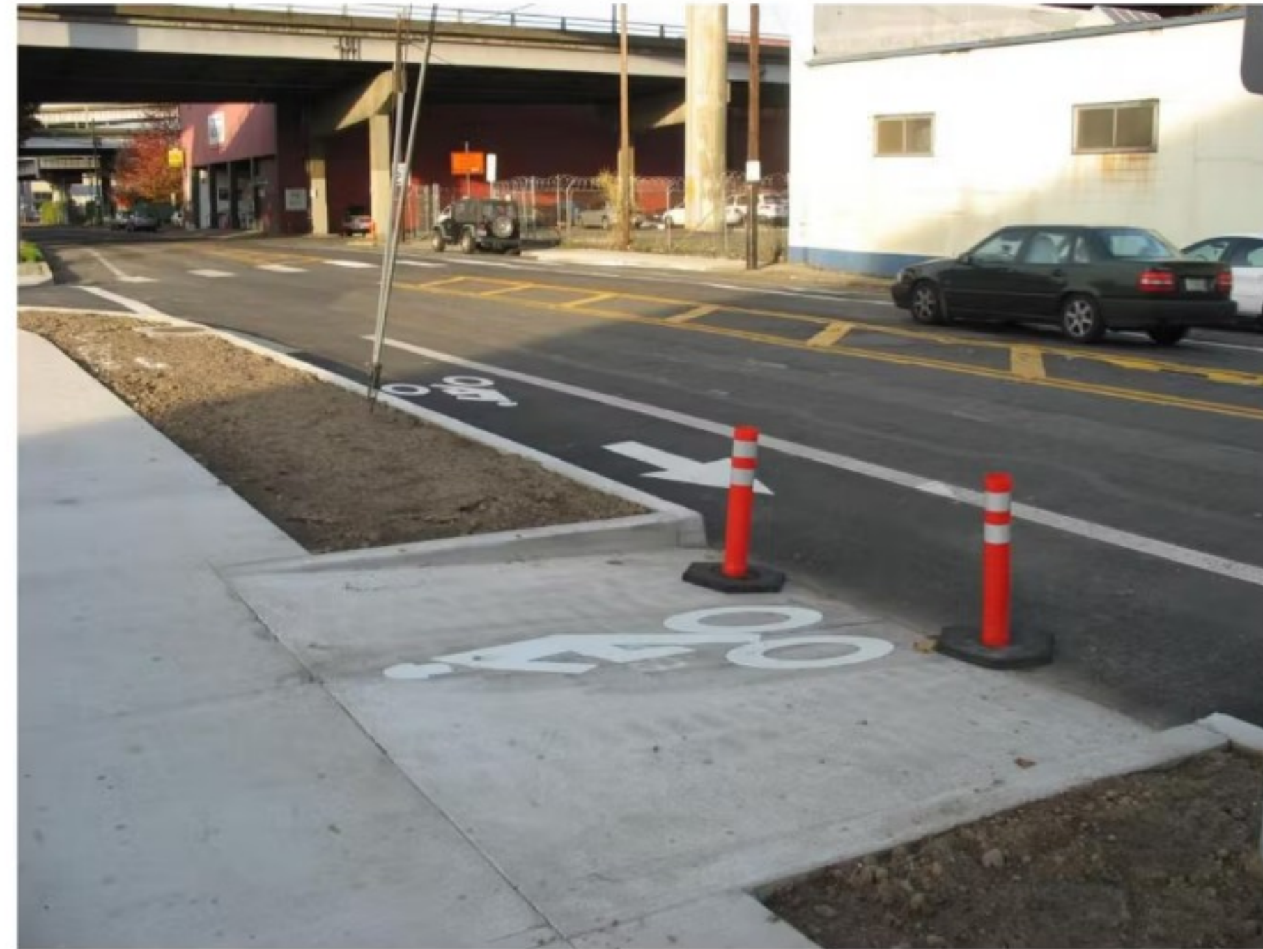
Water Ave bike ramp from Morrison Bridge
