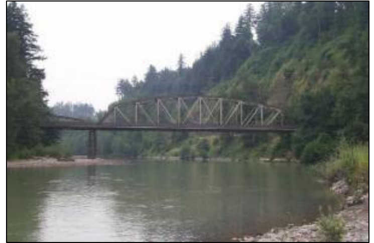
Stark Street Bridge
