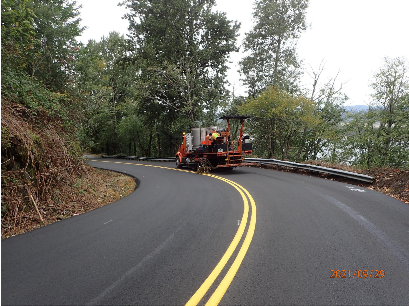
2 nd coat of yellow centerline paint
