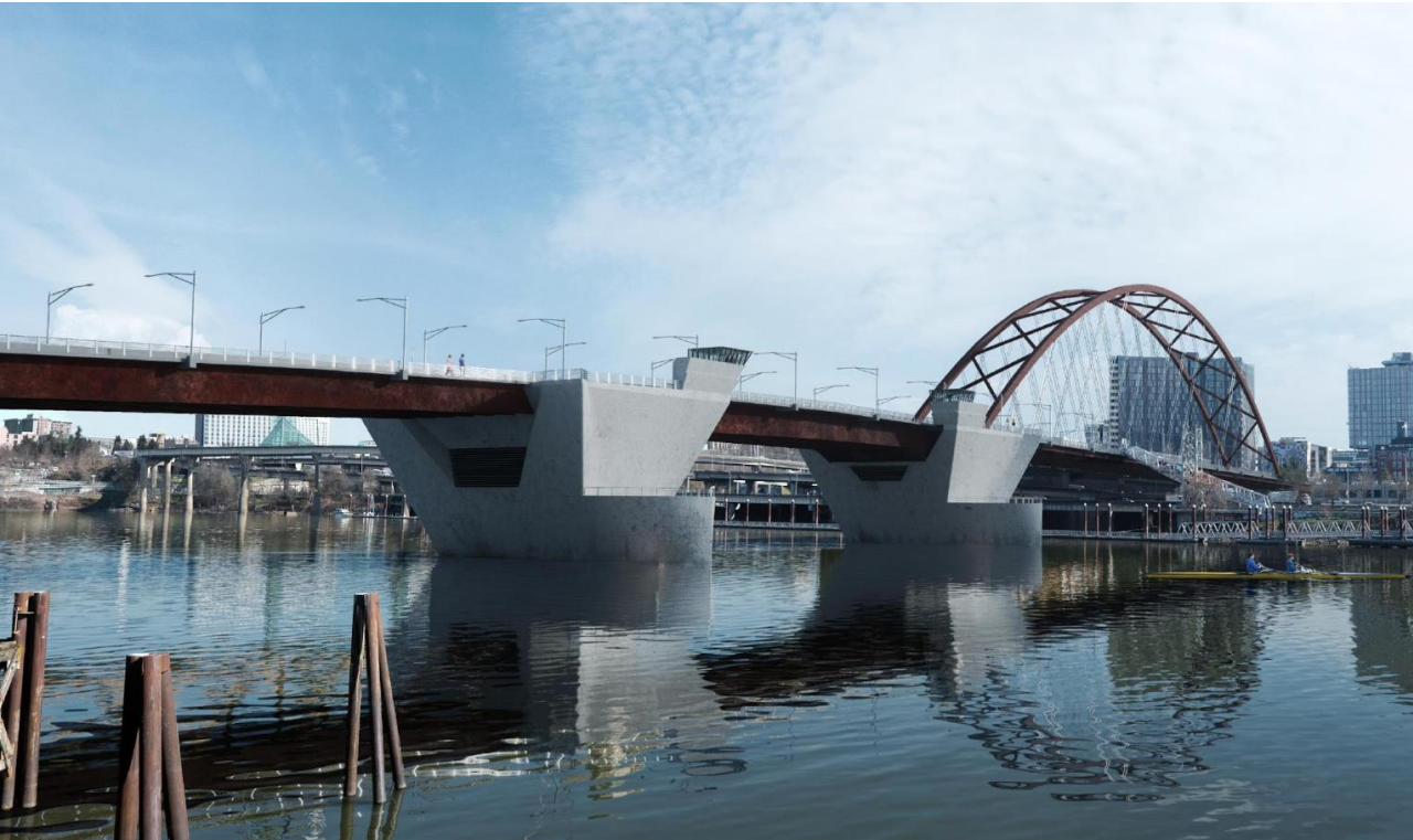
with Tied Arch for eastside long span
