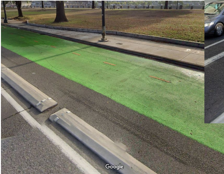
Left Image Description: Photograph showing green bike lanes that are protected by a concrete curb separator
