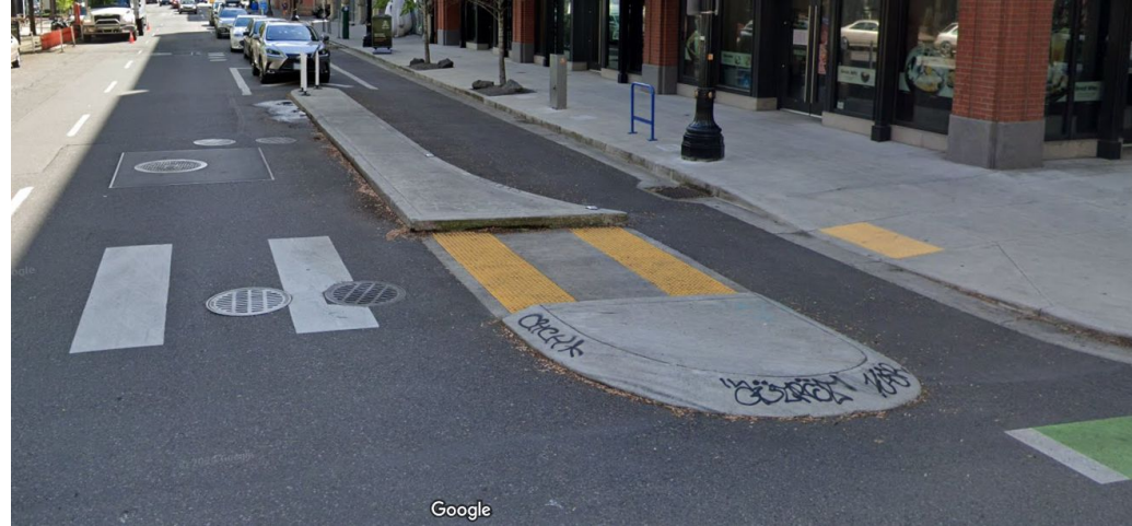
Right Image Description: Photograph showing one concept for a pedestrian refuge, which includes a concrete island for pedestrians to wait between vehicular travel lanes and a bike lane.
