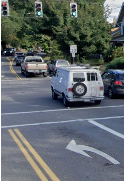
Left Image Description: Photograph showing left turn lane striping and signal head
