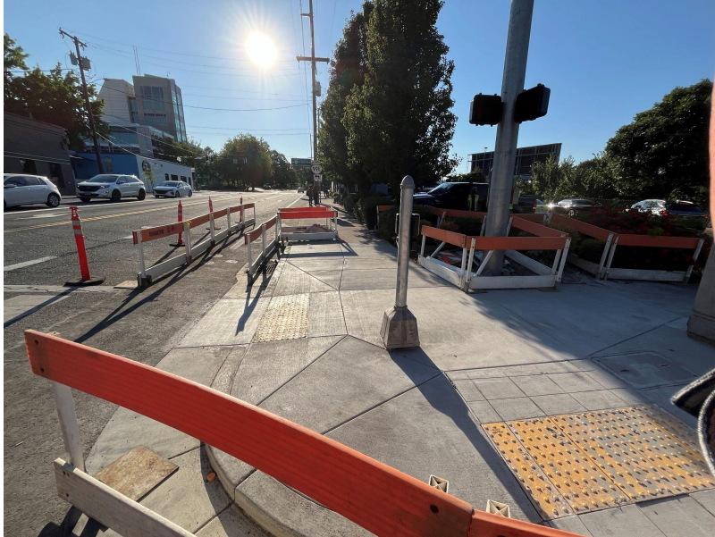
Left Image Description: Photograph showing reconstructed sidewalk, two curb ramps, and a push button pole
