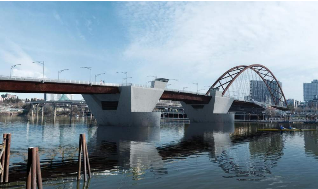
with Tied Arch for eastside long span
