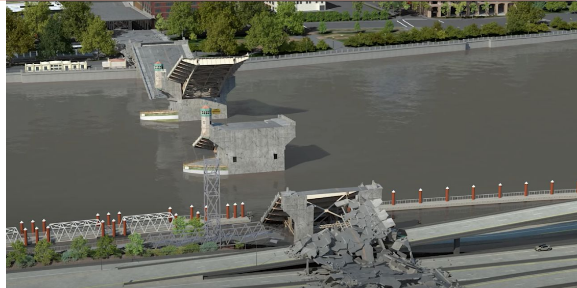
Video: Simulation of Burnside Bridge collapse
